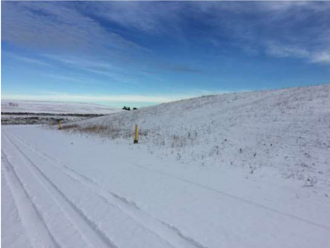
Photo 15- West slope of Cell 1. Slope appears to be in very good condition, well vegetated, no signs of instability or erosion, no woody vegetation, and no observed animal burrows.
