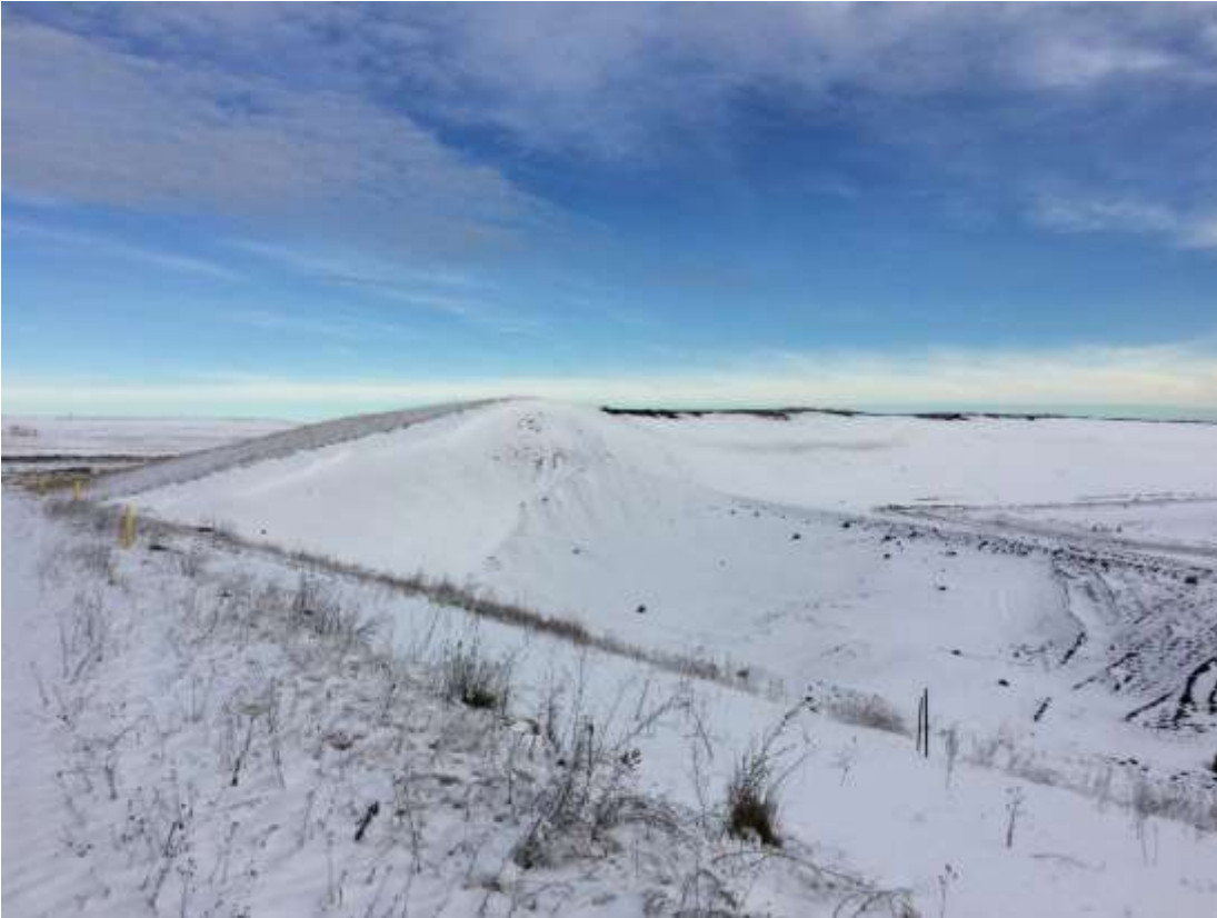
Photo 17- West slope and operational storm water containment ditch. The ditch is in very good condition and prepared for winter and eventual spring runoff
