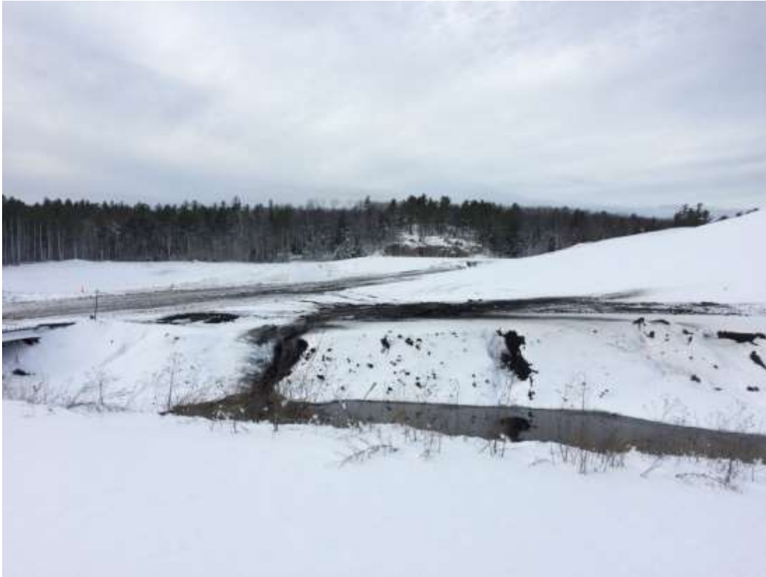
Photo 5- Operational storm water containment ditch north of the entrance, with some minor erosion. The ditch appears to have adequate capacity for the upcoming winter and eventual spring runoff.
