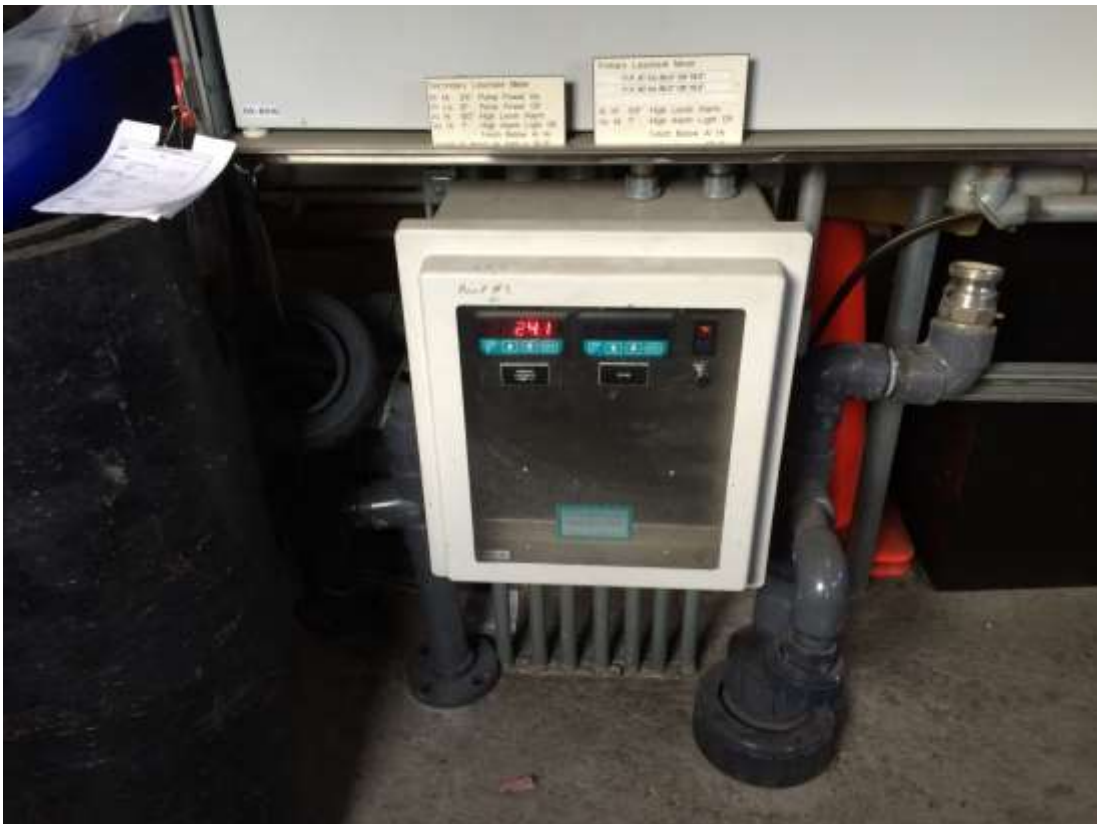
Photo 28- Cell 1 leachate pump controls.
