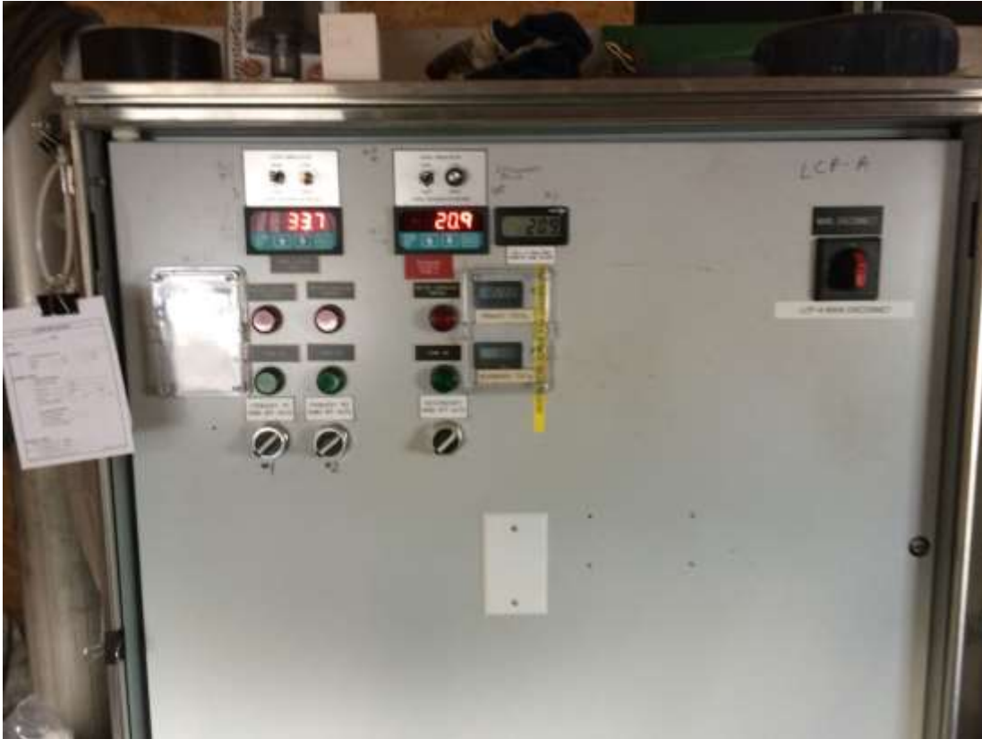
Photo 27- Cell 1 leachate pump controls
