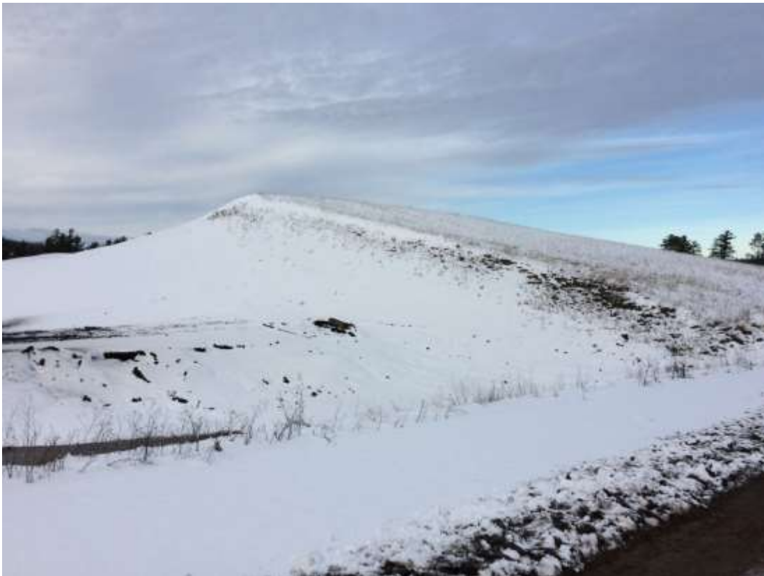
Photo 6- East slope of Cell 1 which was closed in 2014. Slope appears to be in very good condition, well vegetated, no signs of instability or erosion, no woody vegetation, and no observed animal burrows.
