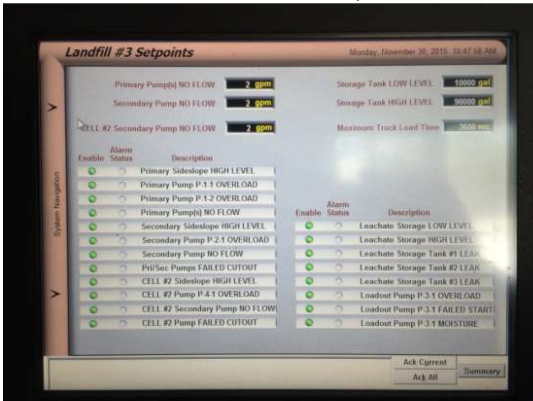
Photo 32 - Landfill No. 3 leachate collection system controls.
