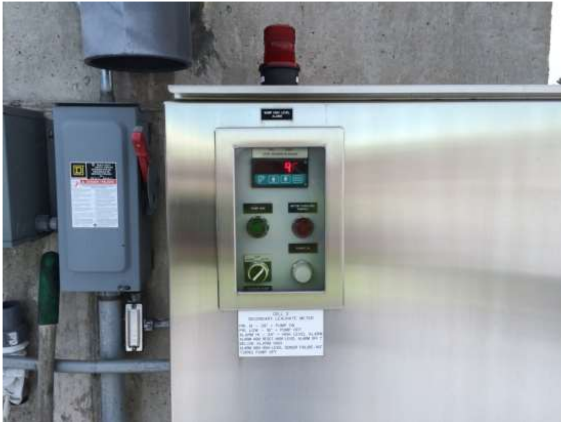
Photo 29- Cell 2 leachate pump controls.
