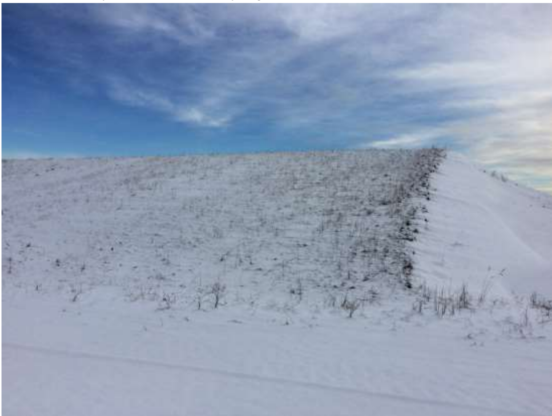
Photo 16 - West slope of Cell 1. Slope appears to be in very good condition, well vegetated, no signs of instability or erosion, no woody vegetation, and no observed animal burrows.
