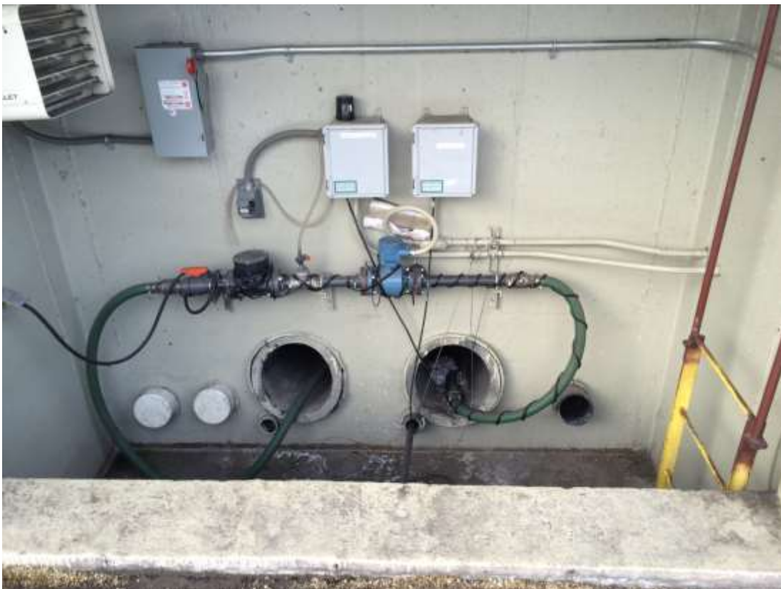
Photo 26- Cell 2 side slope riser vault.
