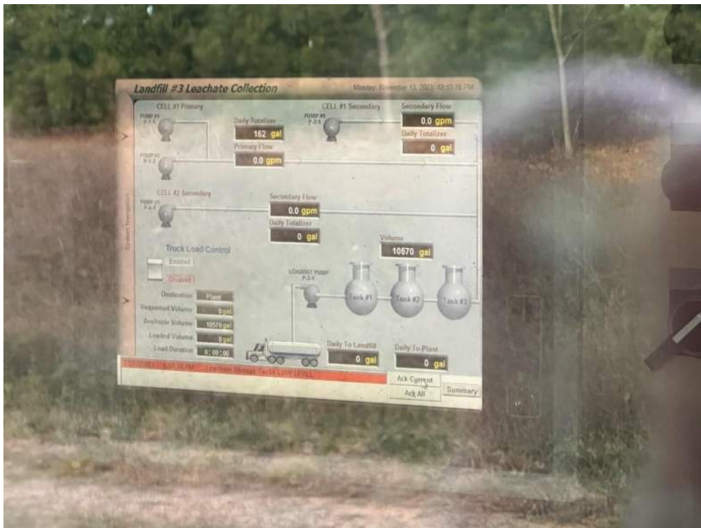
Photo No. 6 – Landfill No. 3 leachate loadout facility screen.
