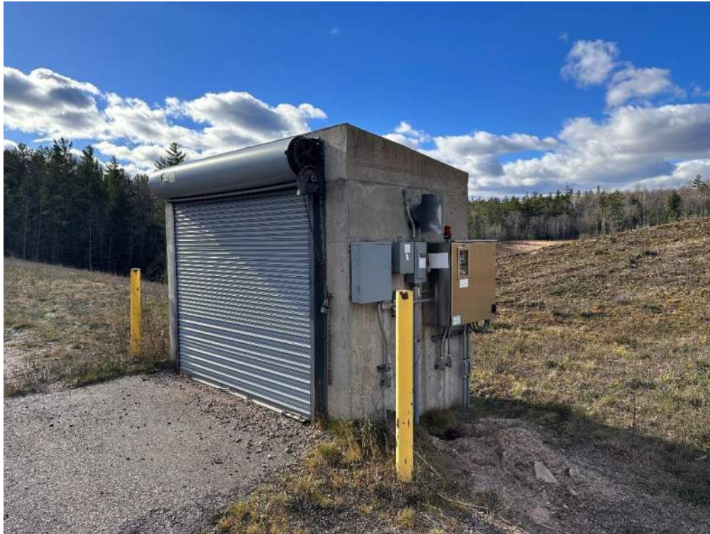
Photo No. 3 – Cell 2 riser vault building
