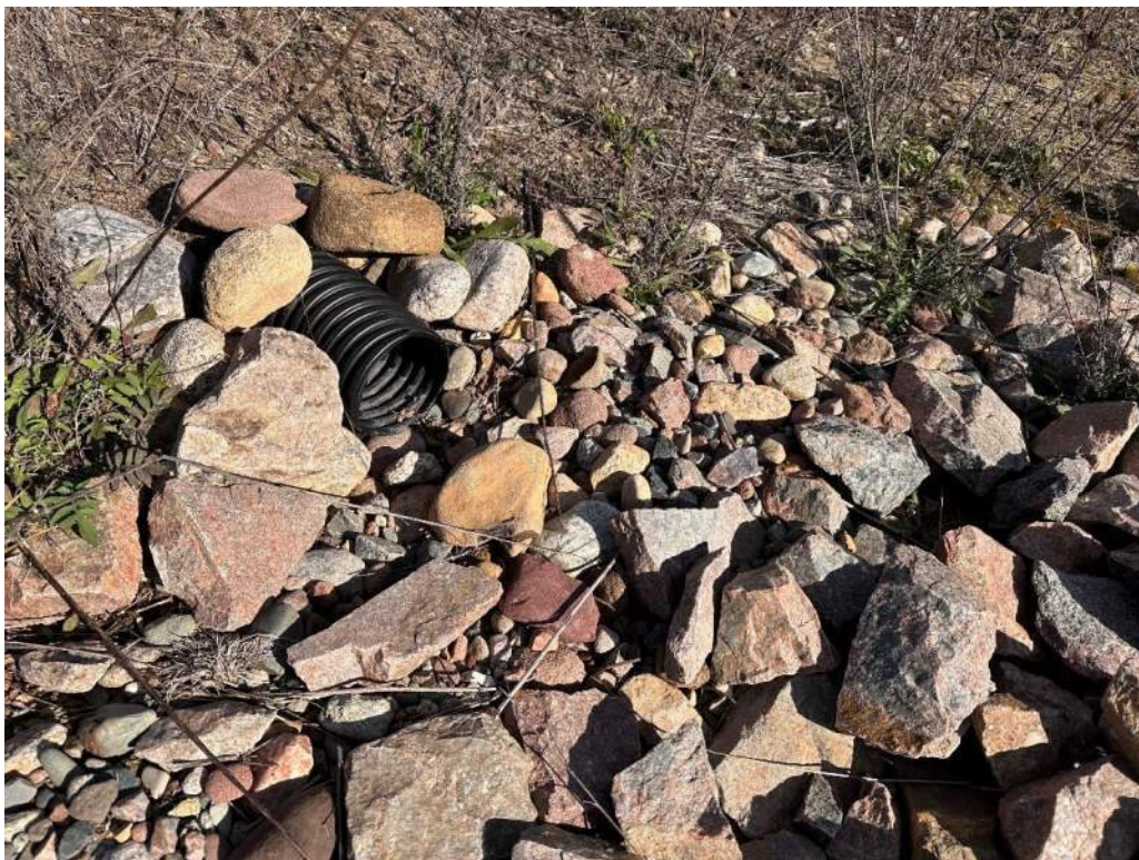
Photo No. 12 – Cover drain outlet located in the borrow area.
