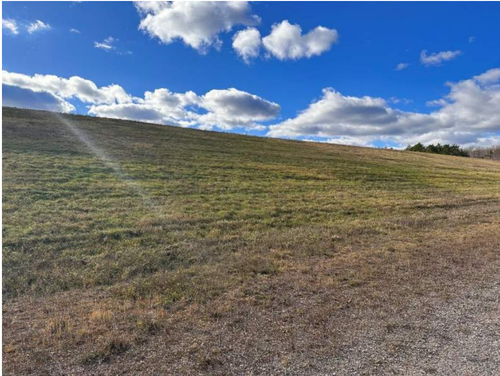
Photo No. 7 – North slope of Landfill No. 3, looking south.
