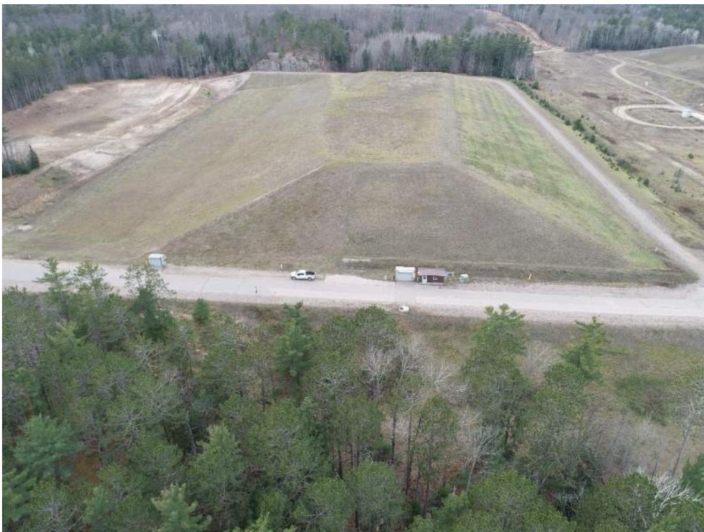
Photo No. 16 – Landfill No. 3, looking west.
