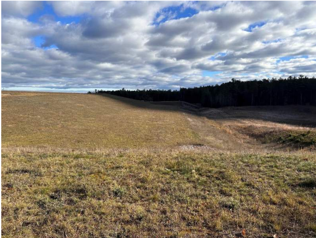
Photo No. 11 – South slope of Landfill No. 3, looking east.
