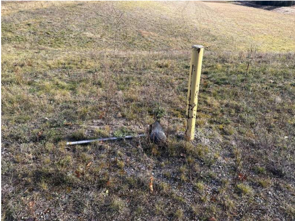
Photo No. 13 – Leachate cleanout on the west side of Landfill No. 3.
