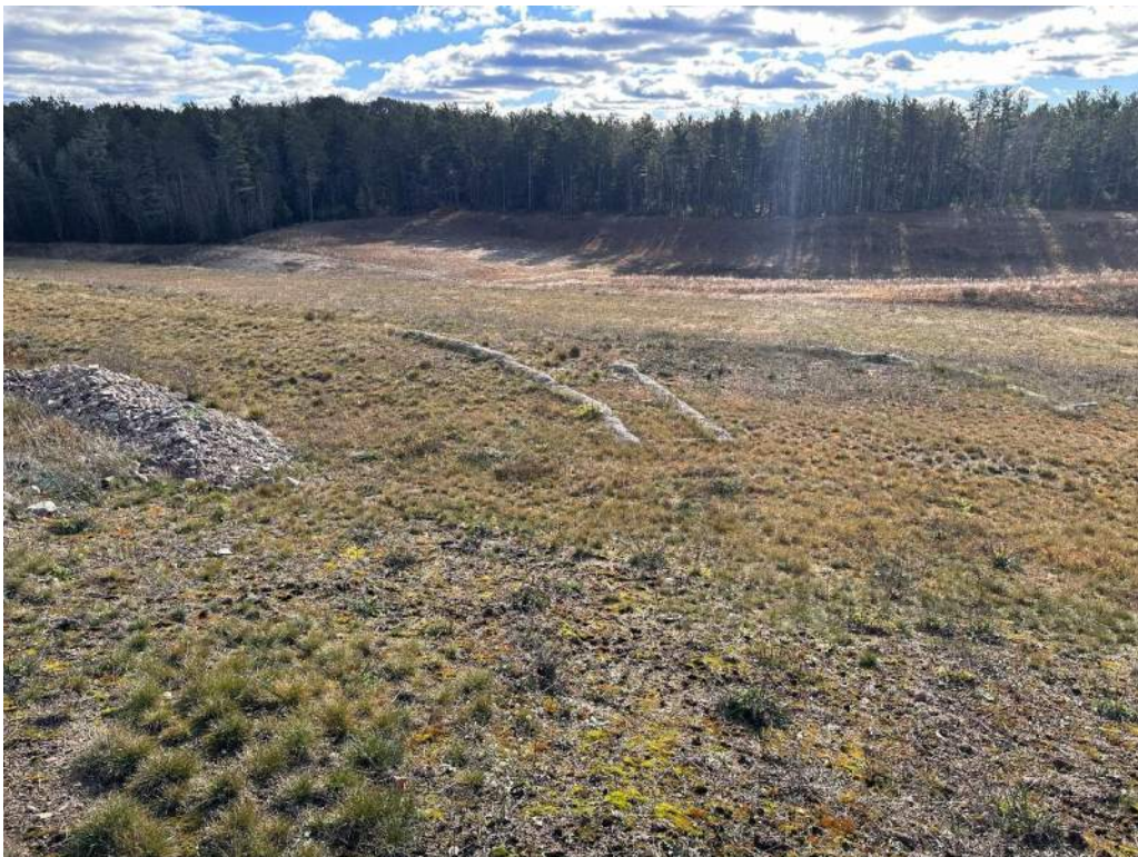
Photo No. 10 – Cover erosion control berms.
