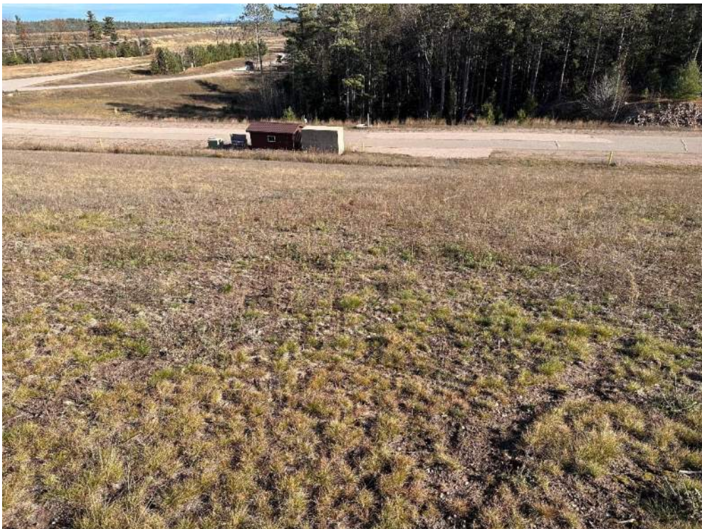
Photo No. 4 – Cell 1 east slope and riser vault building.
