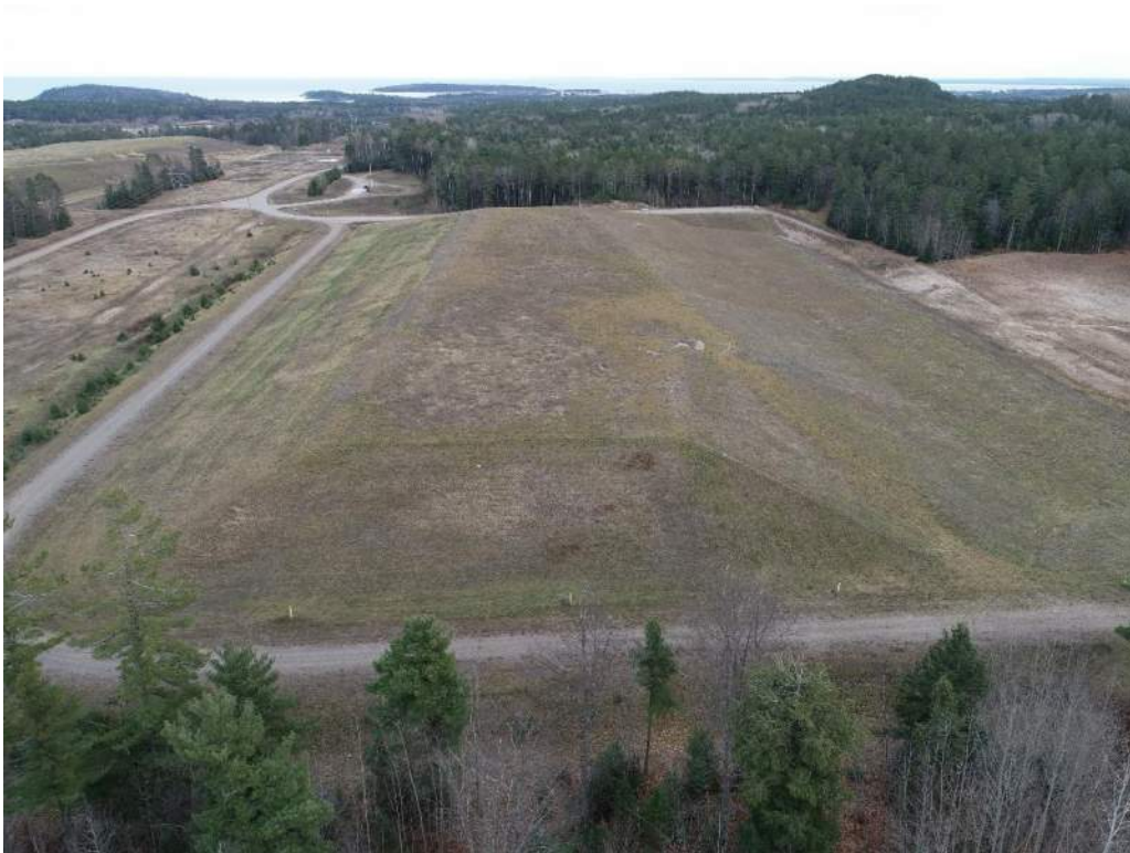
Photo No. 15 – Landfill No. 3, looking east.
