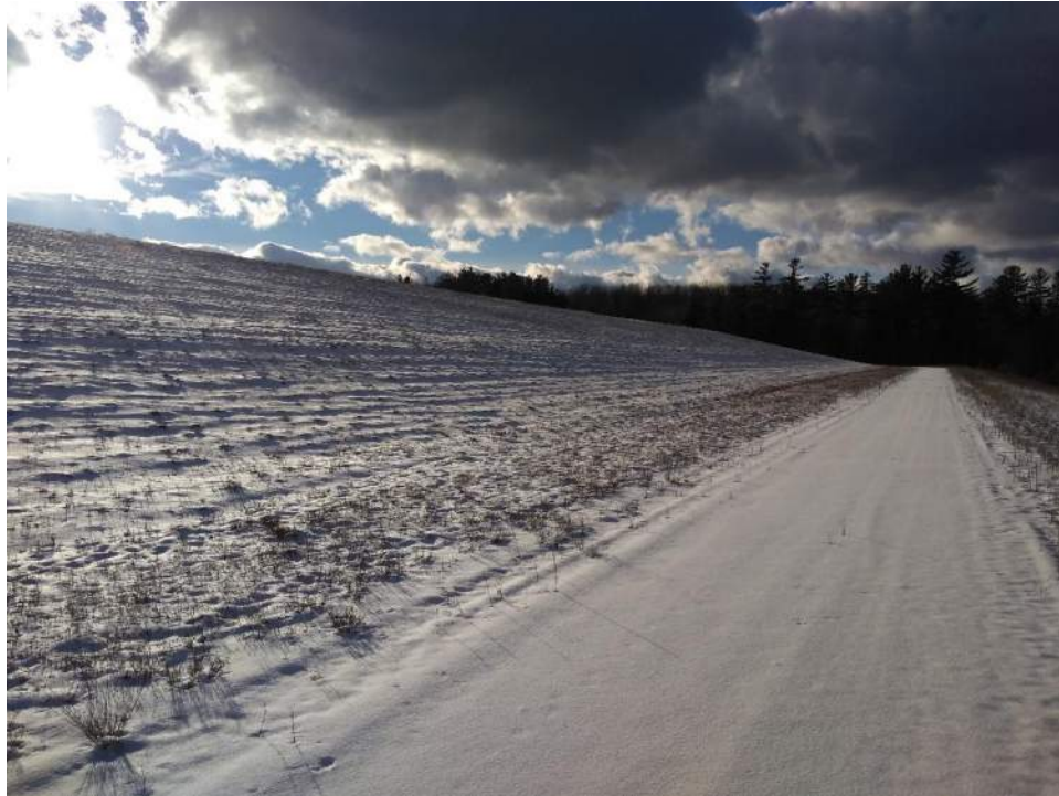
Photo No. 1: Toe of north slope of the PIPP Landfill No. 3, looking west.
