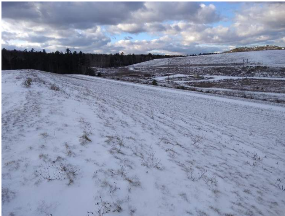
Photo No. 2: Top of north slope, looking northwest
