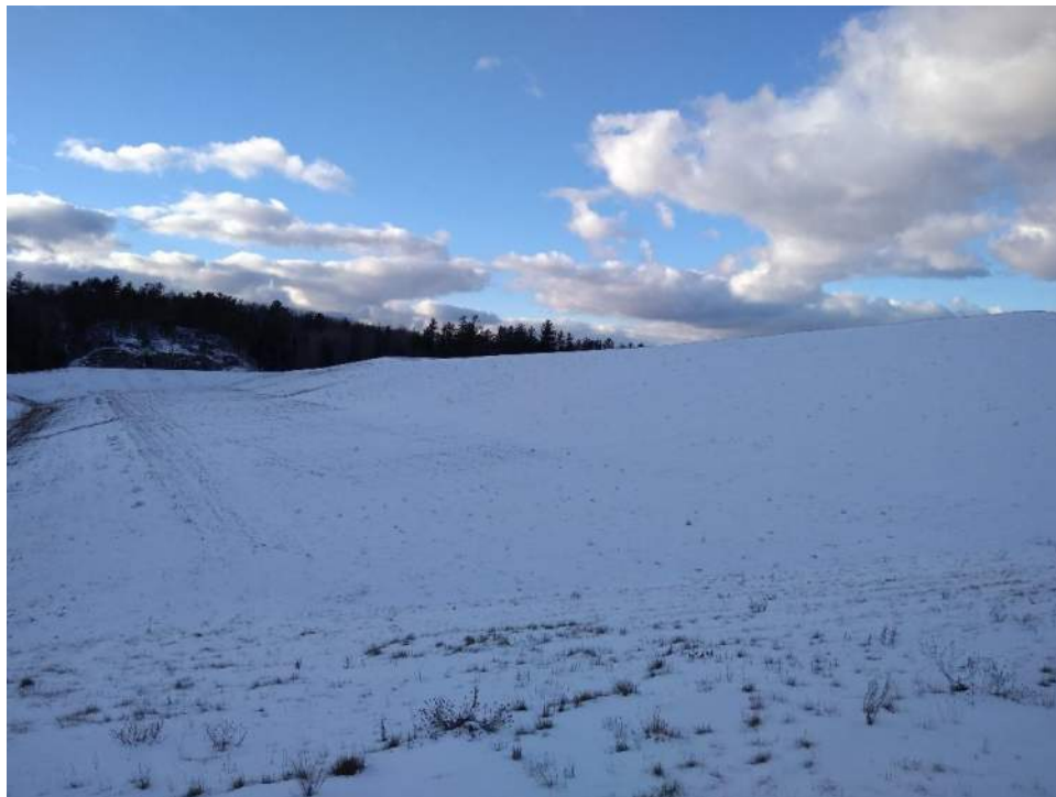
Photo No. 8: South slope of the PIPP Landfill No. 3 looking west.
