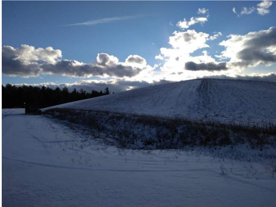
Photo No. 9: East slope of the PIPP Landfill No. 3 looking south.
