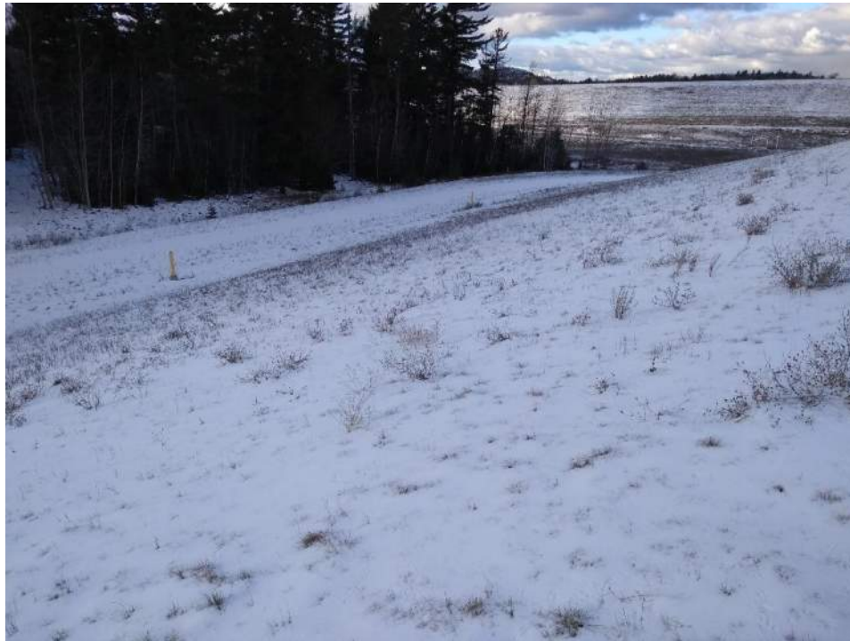
Photo No. 3: West slope of the PIPP Landfill No. 3 looking north.
