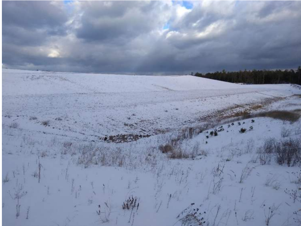
Photo No. 7: South slope of the PIPP Landfill No. 3 looking northeast.
