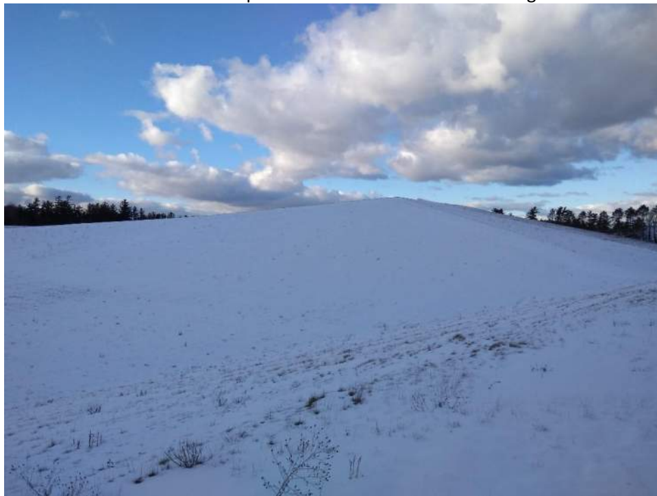
Photo No. 10: East slope of the PIPP Landfill No. 3 looking northwest.
