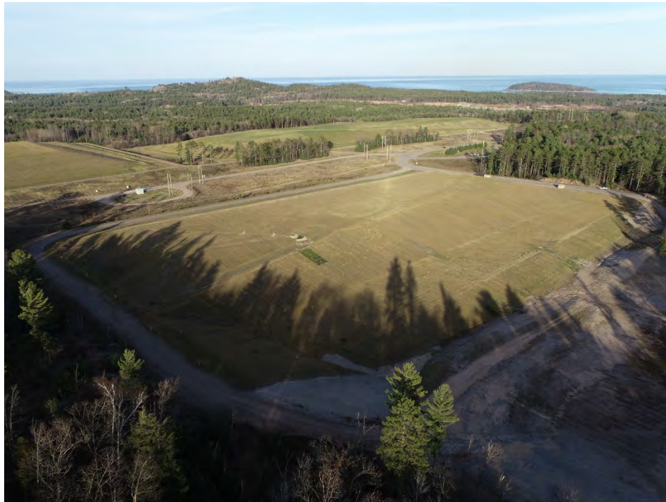
Photo No. 1: Aerial photo of PIPP Landfill No. 3 looking northeast 11/6/2020
