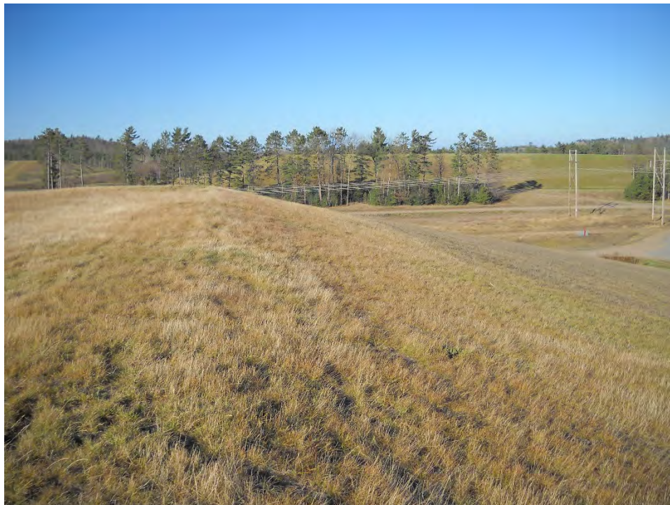
Photo No. 4: East slope of the PIPP Landfill No. 3 looking north 11/4/2020
