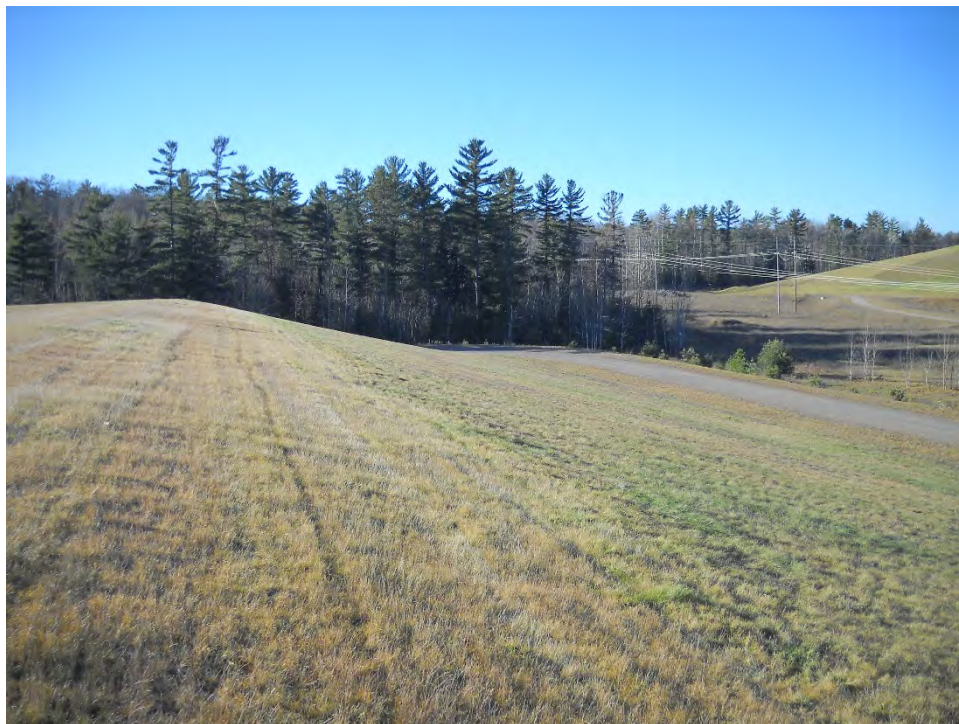
Photo No. 8: North slope of the PIPP Landfill No. 3 looking west 11/4/2020
