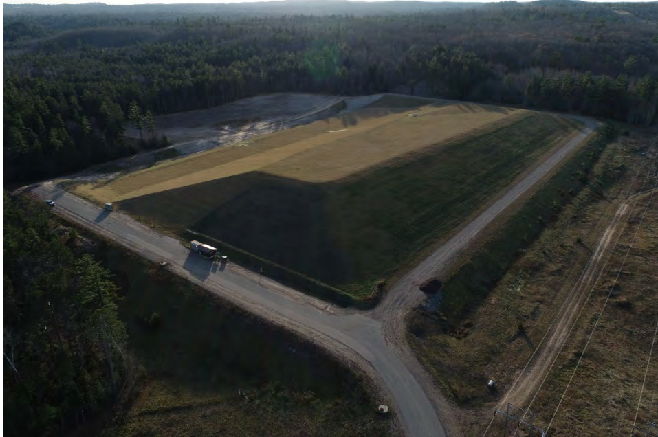
Photo No. 5: East and north slopes of the PIPP Landfill No. 3 looking southwest 11/6/2020
