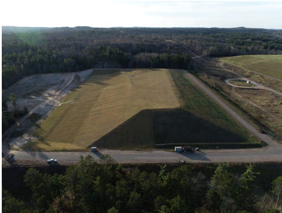
Photo No. 3: East slope of the PIPP Landfill No. 3 looking west 11/6/2020
