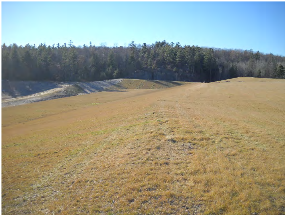
Photo No. 2: South slope of the PIPP Landfill No. 3 looking west 11/4/2020
