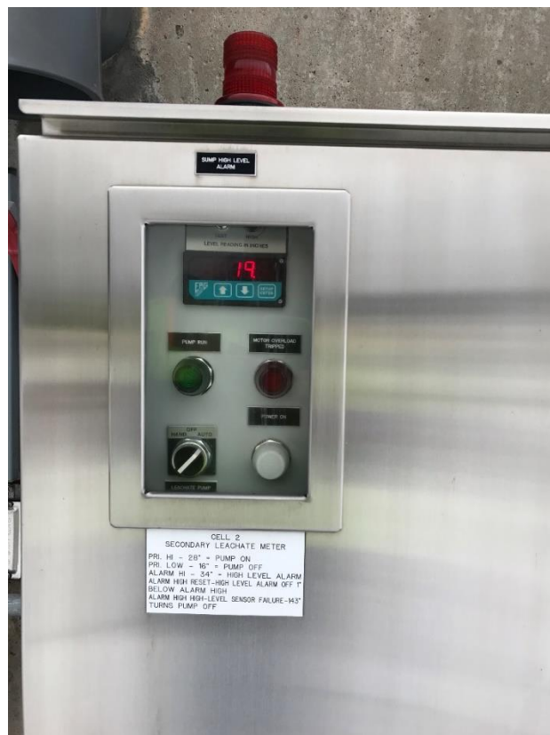
Photo 12 – Cell 2 leachate pump controls.
