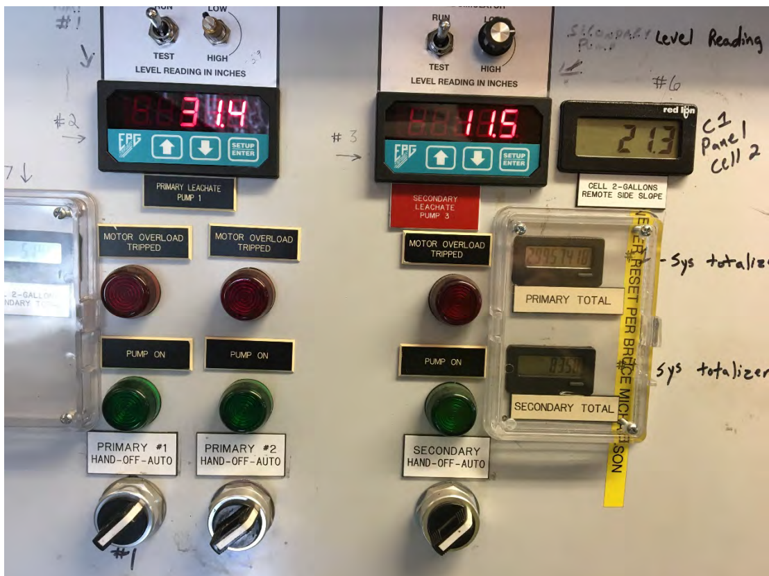
Photo 15 – Cell 1 leachate pump controls.
