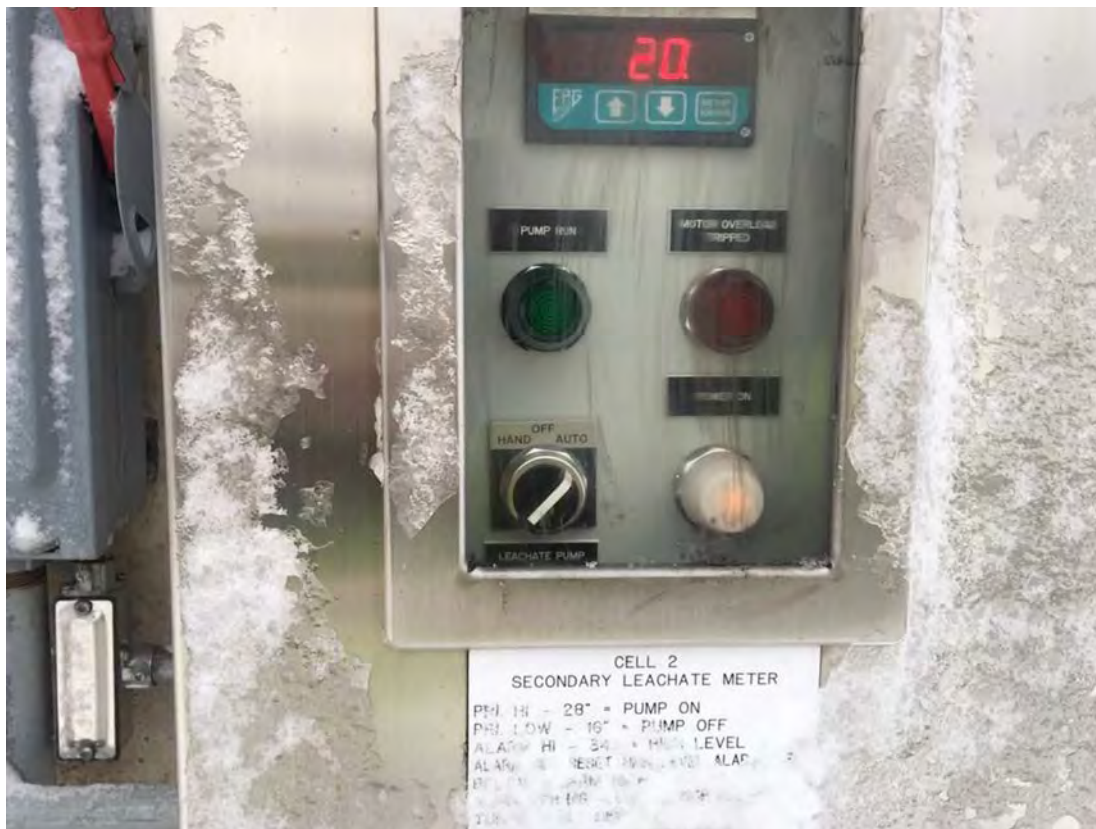
Photo 17 – Cell 2 leachate pump controls.
