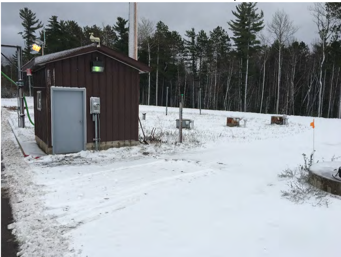
Photo 12 – Leachate load out building and leachate tank risers.
