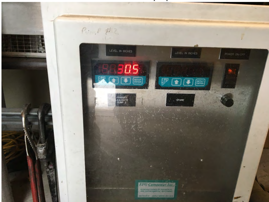
Photo 16 – Cell 1 leachate pump controls.
