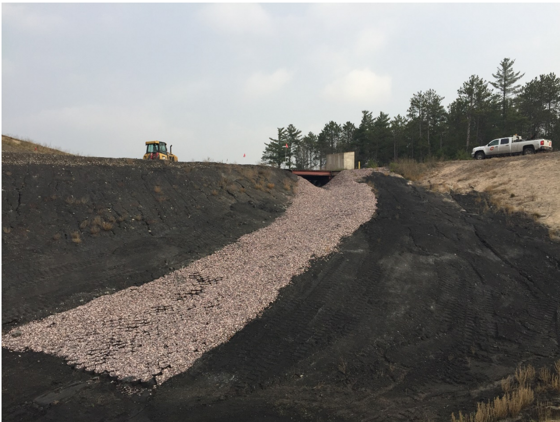
Photo 20 – View of temporary erosion protection of ash at cell entrance and cattle guard.
