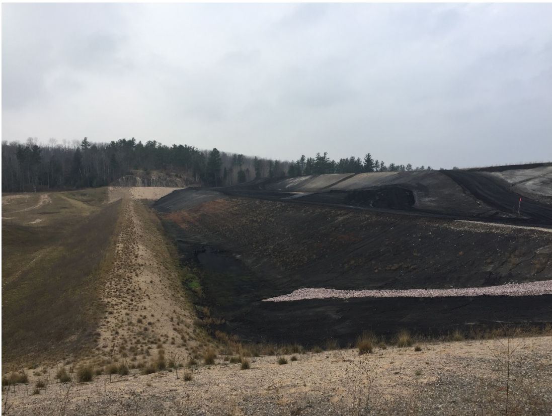
Photo 4- Looking west at the south containment berm and operational storm water containment area. The operational storm water containment area is graded as required by the design.
