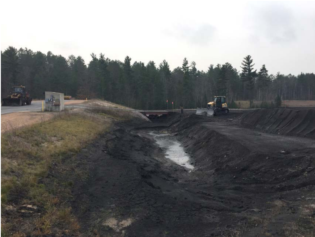
Photo 5- Operational storm water containment ditch north of the entrance. The ditch was recently cleaned out and in the process of regrading in preparation for winter and eventual spring runoff.
