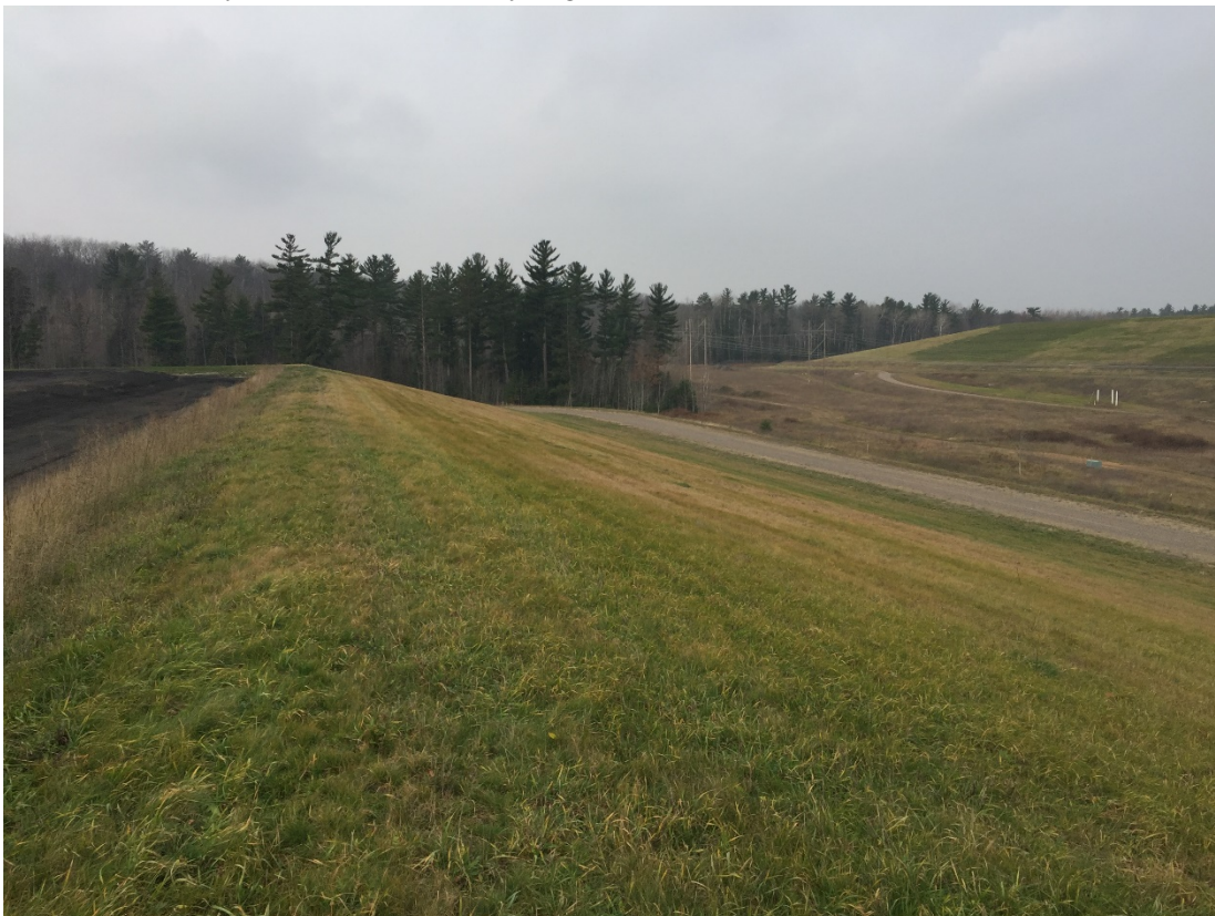
Photo 12- - North Slope of Cell 1. Slope appears to be in very good condition, well vegetated, no signs of instability or erosion, no woody vegetation, and no observed animal burrows.
