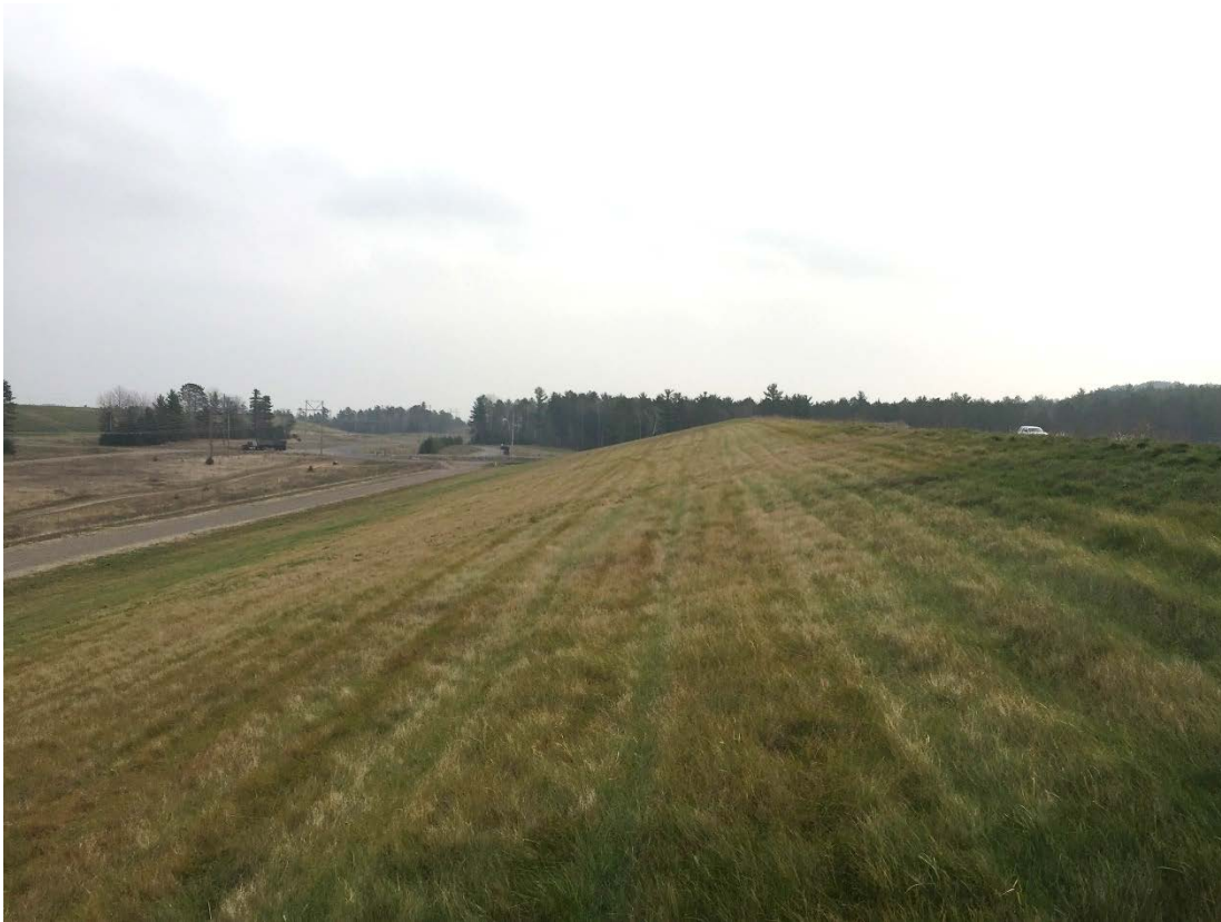
Photo 13- - North Slope of Cell 1. Slope appears to be in very good condition, well vegetated, no signs of instability or erosion, no woody vegetation, and no observed animal burrows.
