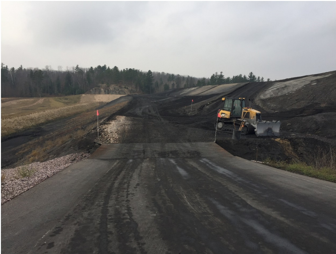
Photo 3- Entrance into Cell 2 looking west at cattle crossing used for storm water and track-out control.
