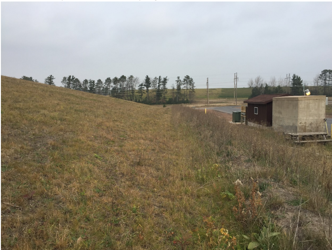
Photo 8- East Slope of Cell 1. Slope appears to be in very good condition, well vegetated, no signs of instability or erosion, no woody vegetation, and no observed animal burrows.
