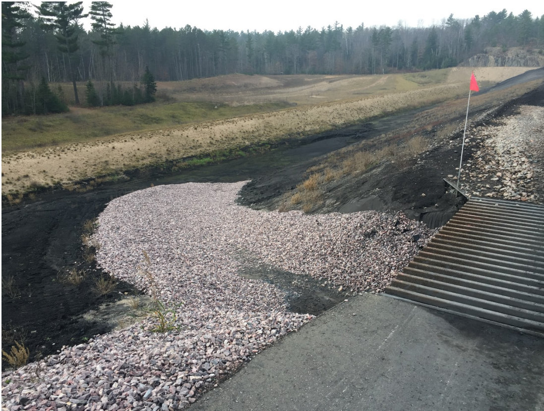
Photo 19 – View of temporary erosion protection installed to protect cell entrance road and cattle guard.
