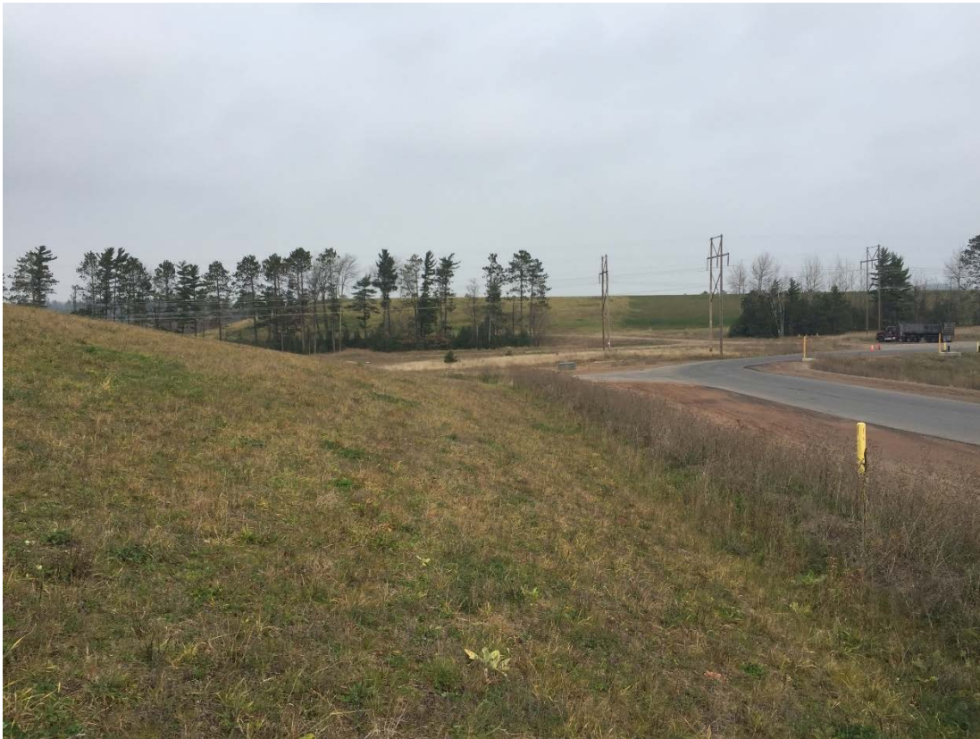
Photo 9- East Slope of Cell 1. Slope appears to be in very good condition, well vegetated, no signs of instability or erosion, no woody vegetation, and no observed animal burrows.
