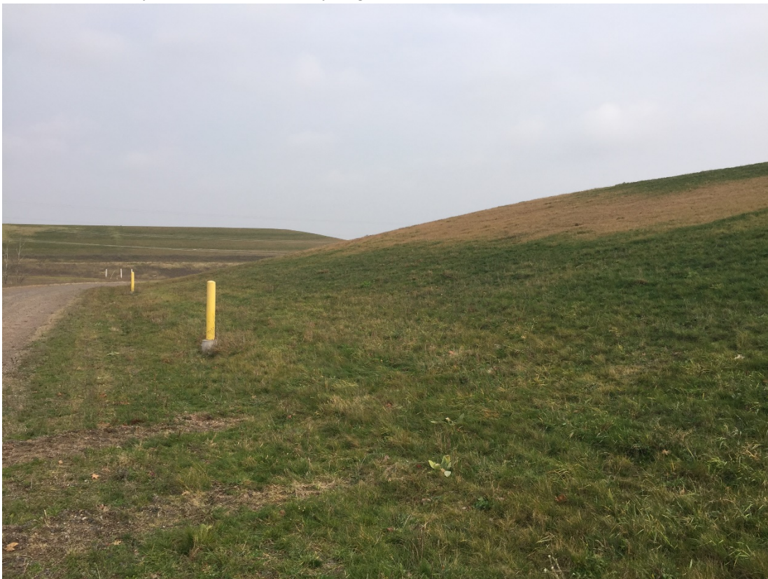
Photo 14 - West Slope of Cell 1. Slope appears to be in very good condition, well vegetated, no signs of instability or erosion, no woody vegetation, and no observed animal burrows.
