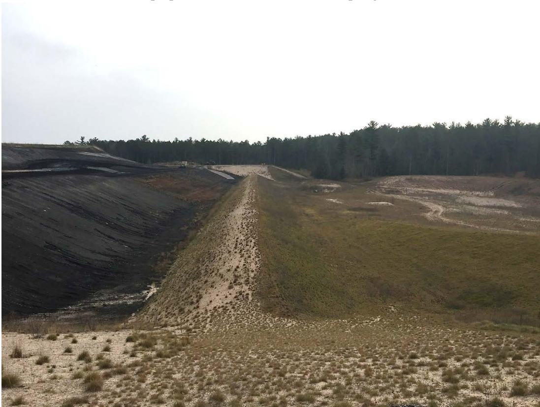
Photo 16 - Looking east at the south containment berm and operational storm water containment area. The operational storm water containment area is graded as required by the design.
