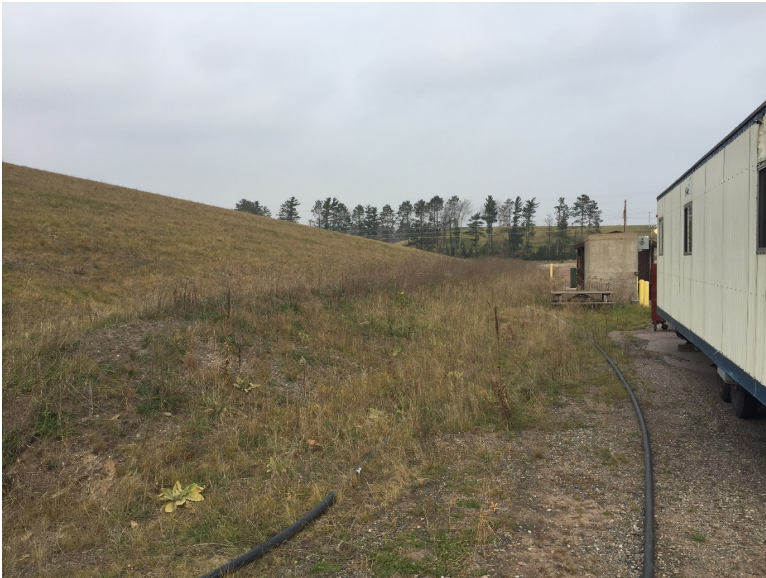
Photo 7- East Slope of Cell 1. Slope appears to be in very good condition, well vegetated, no signs of instability or erosion, no woody vegetation, and no observed animal burrows.
