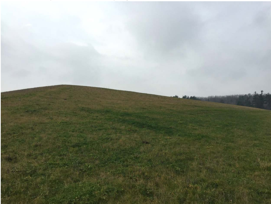
Photo 11- East Slope of Cell 1. Slope appears to be in very good condition, well vegetated, no signs of instability or erosion, no woody vegetation, and no observed animal burrows.
