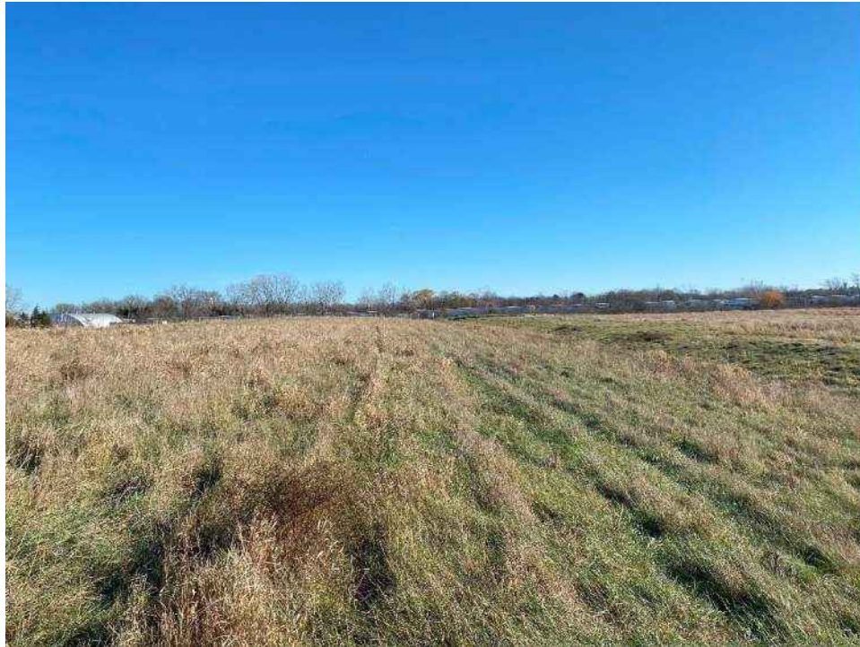
Photo No. 5 – South slope of Cell 1 and perimeter stormwater ditch, looking east.
