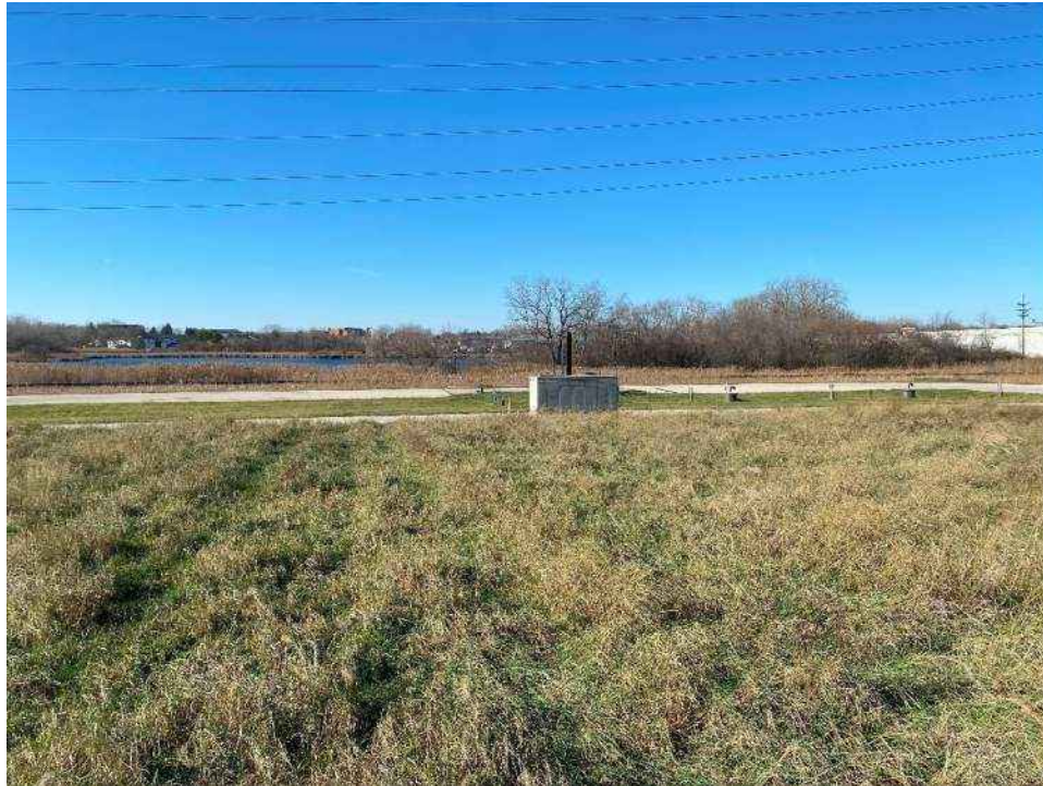
Photo No. 3 – Looking west from the Cell 1 cover at the leachate loadout pad.
