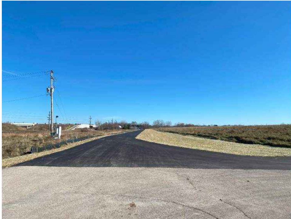
Photo No. 9 – Southwest corner of Cell 1 cover, looking east.
