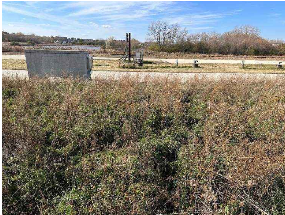
Photo No. 3 – Looking west from the Cell 1 cover at the leachate loadout pad.
