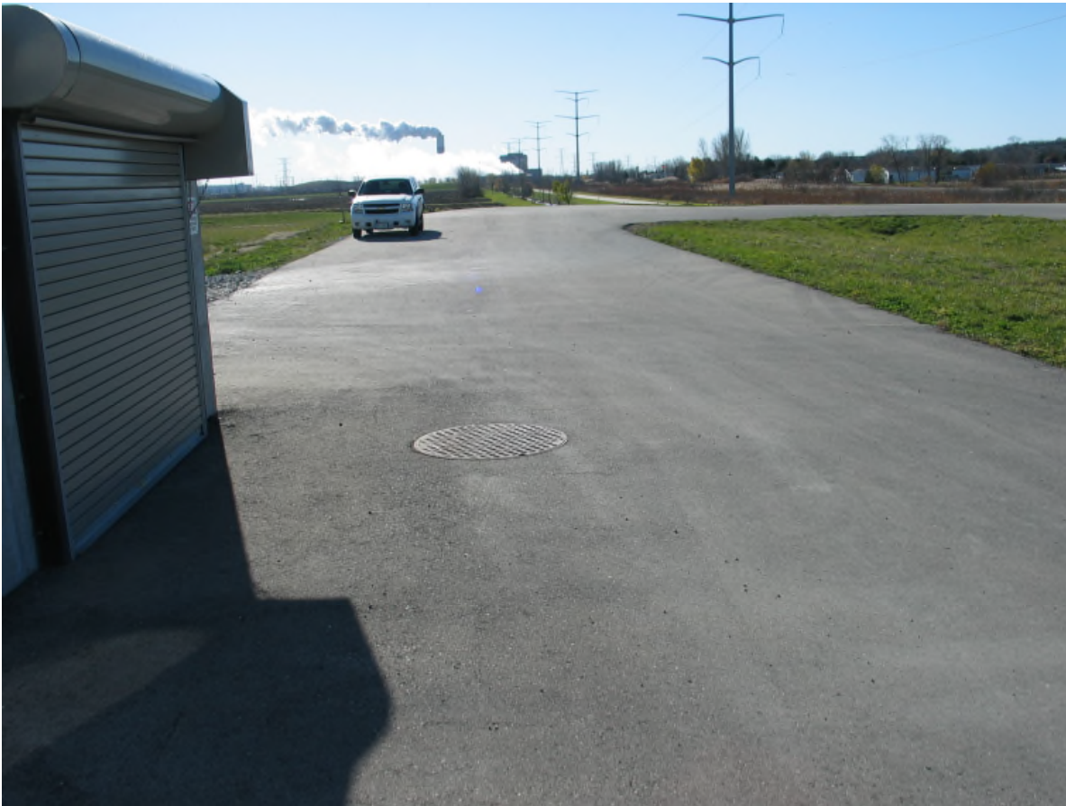
Access Road at Riser Vault (looking south)
