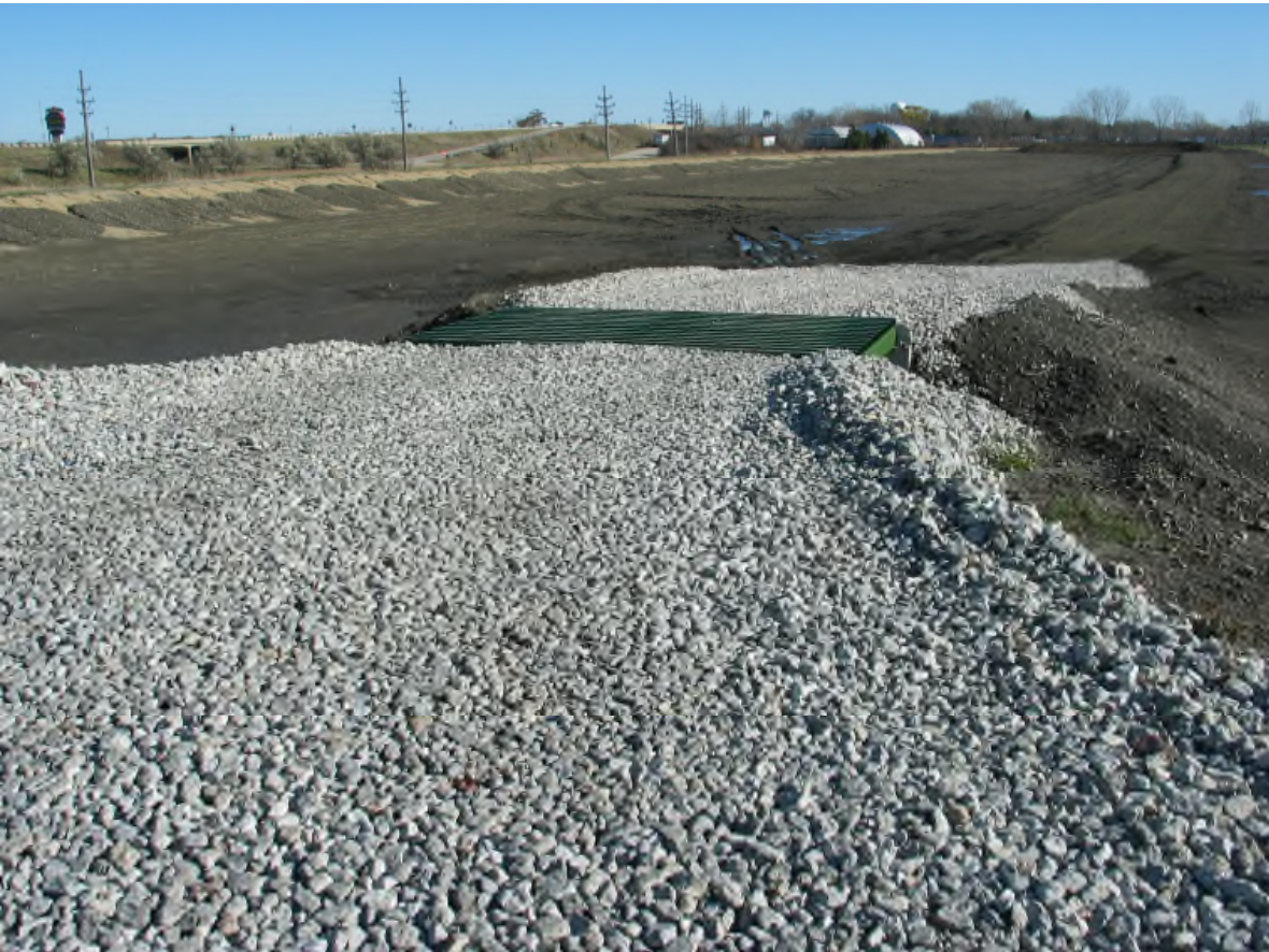
Cell Entrance (looking east)
