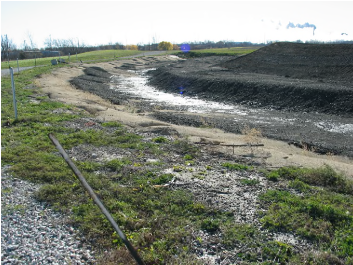
East Perimeter Berm (looking south)
