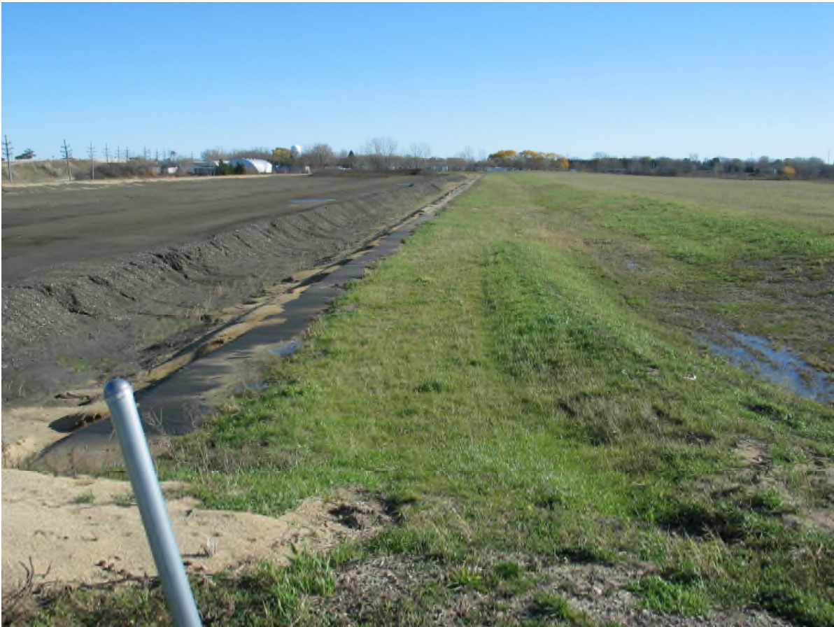
Intercell (South) Berm (looking east)
