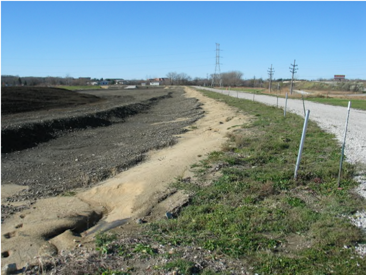
North Perimeter Berm (looking west)
