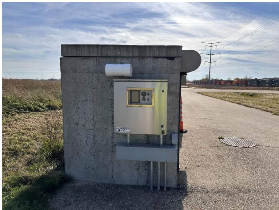
Photo No. 2 – Leachate sump collection vault.
