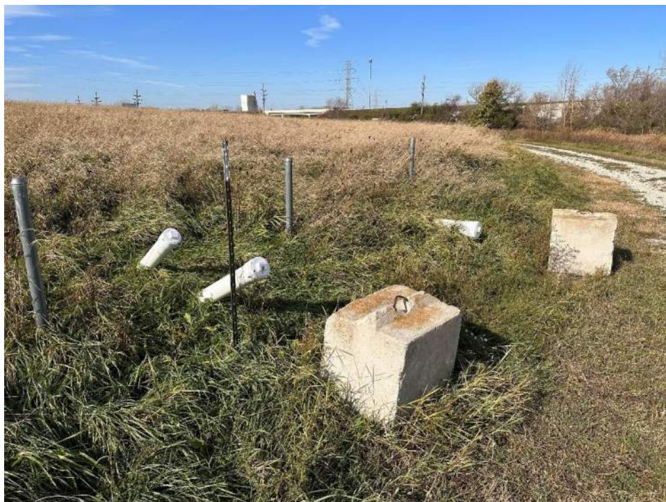
Photo No. 6 – Cleanout and leachate headwell on the east end of Cell 1.
