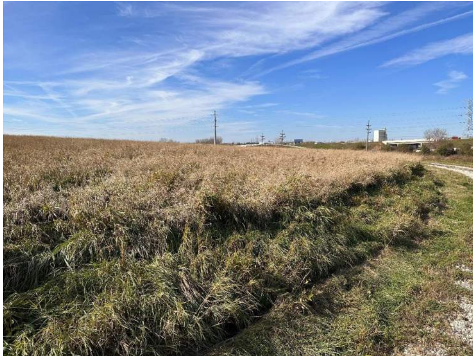
Photo No. 5 – East slope of Cell 1, looking northwest.
