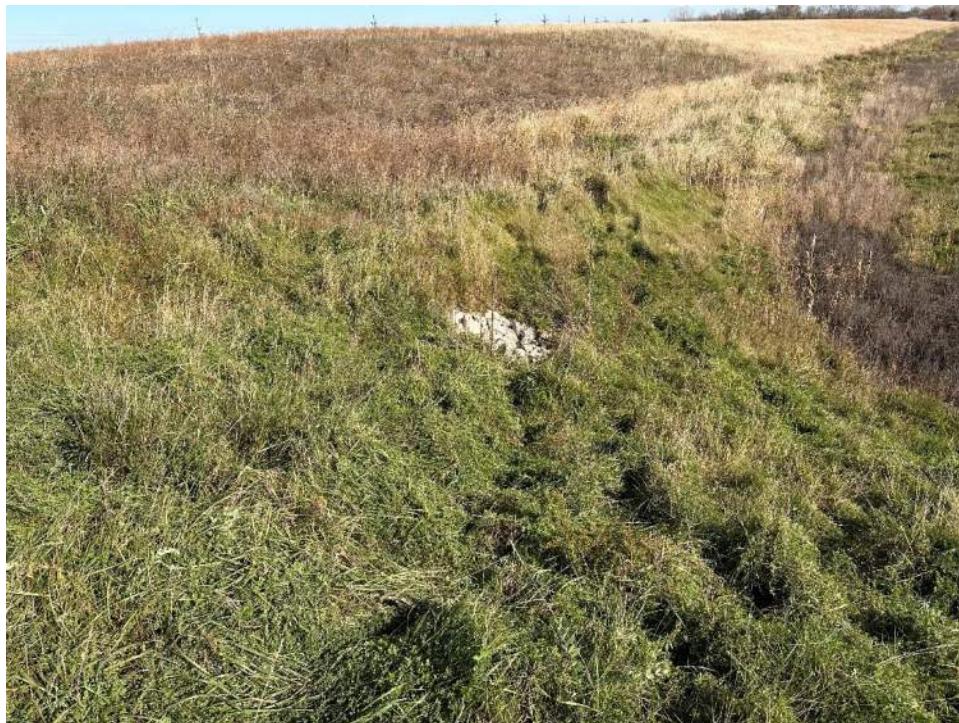
Photo No. 8 – Final cover drain pipe outlet on the south slope.
