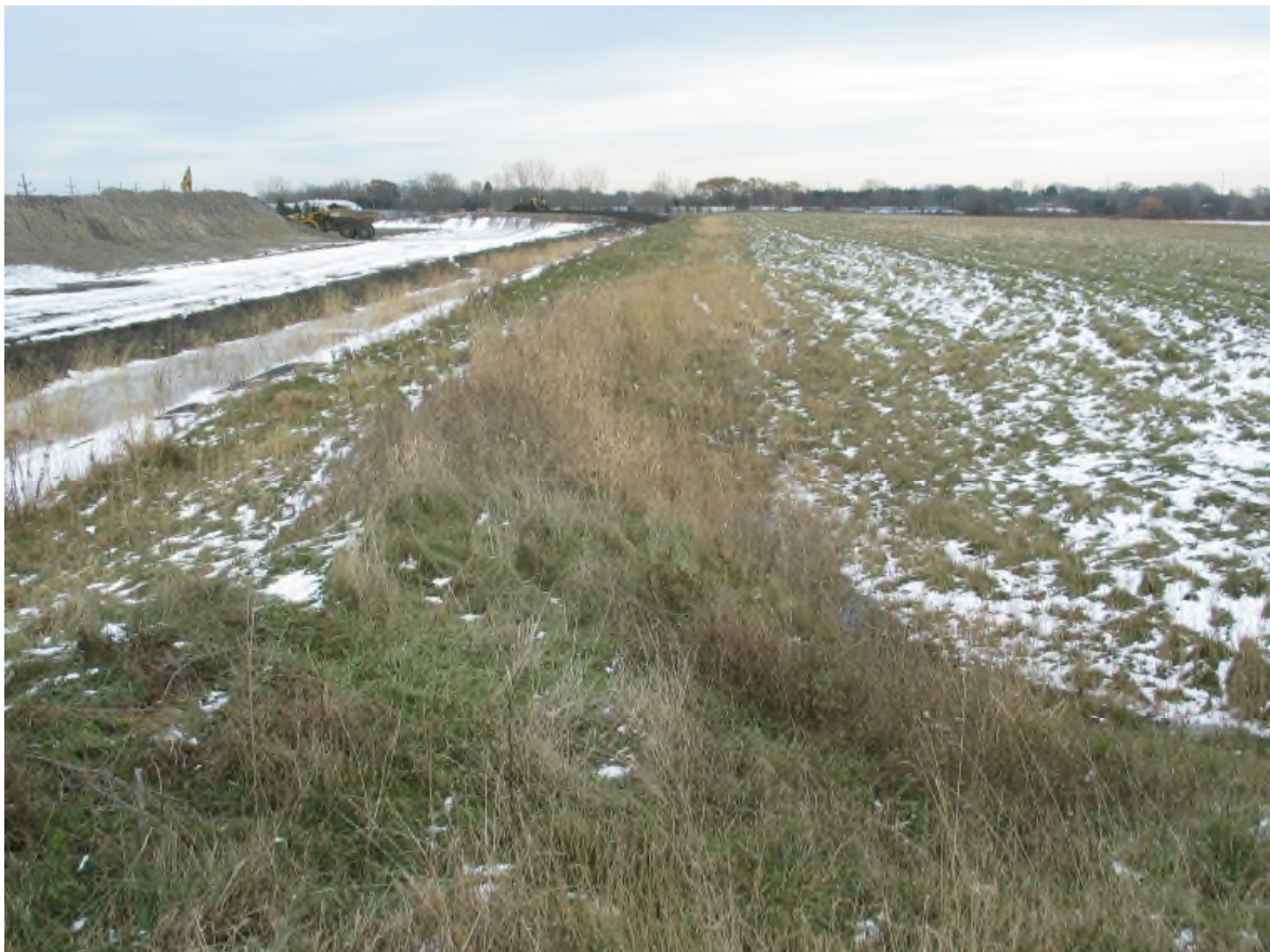
West End Intercell Berm (looking east)
