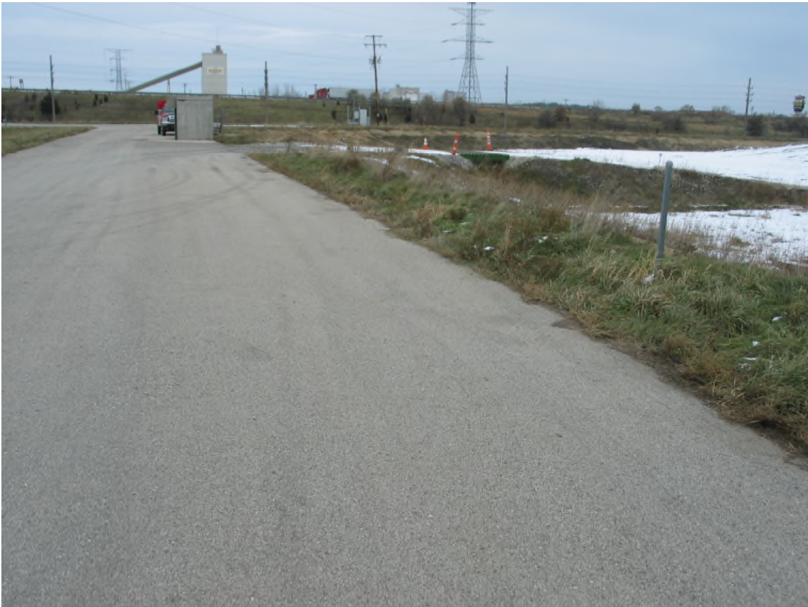
Access Road and Cell Entrance (looking north)
