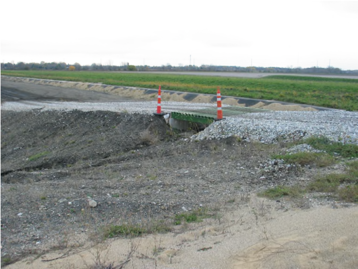
Cell Entrance (looking southeast)
