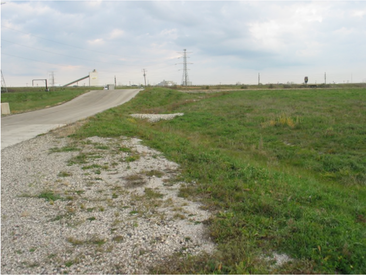
Access Road & Surface Water Ditch (looking north)
