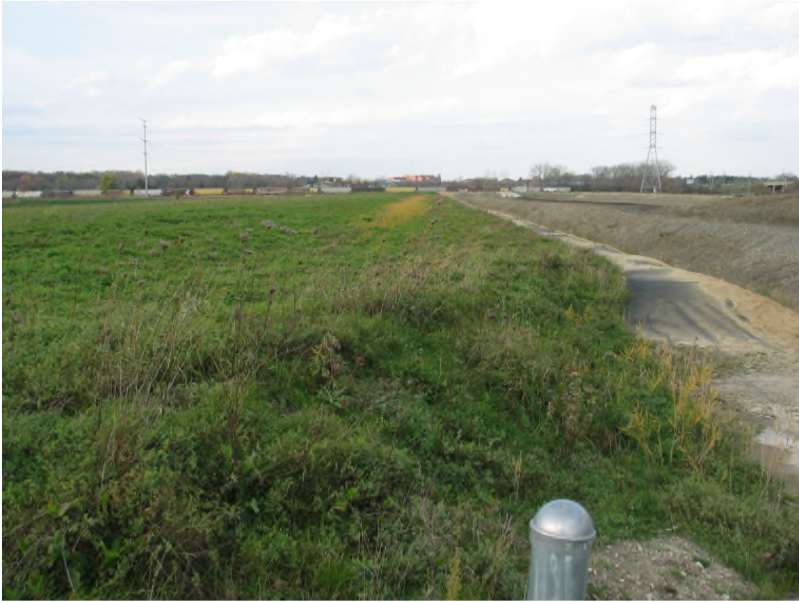
East End Intercell Berm Berm (looking west)
