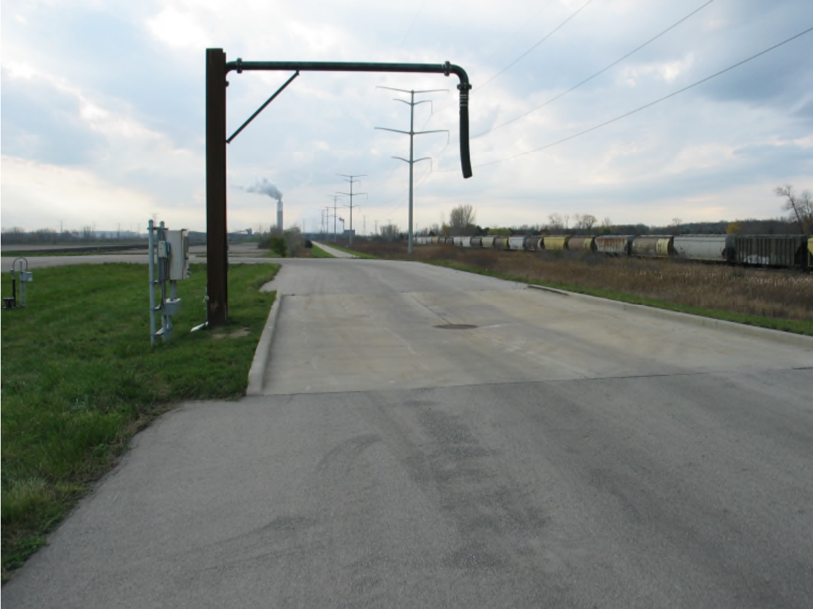
Leachate Loadout Pad (looking south)
