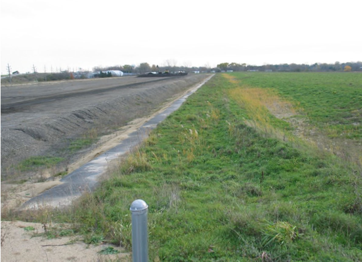
West End Intercell Berm (looking east)
