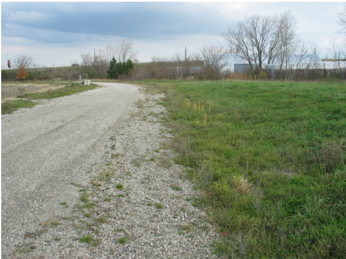
Cell 1 East Berm (looking north)
