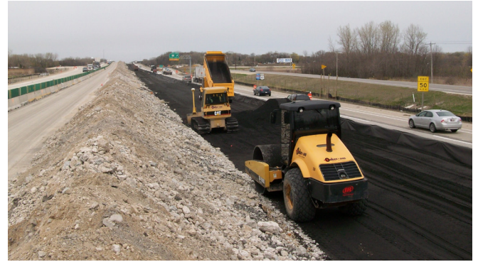
I-94 reconstruction with bottom ash sub-base
