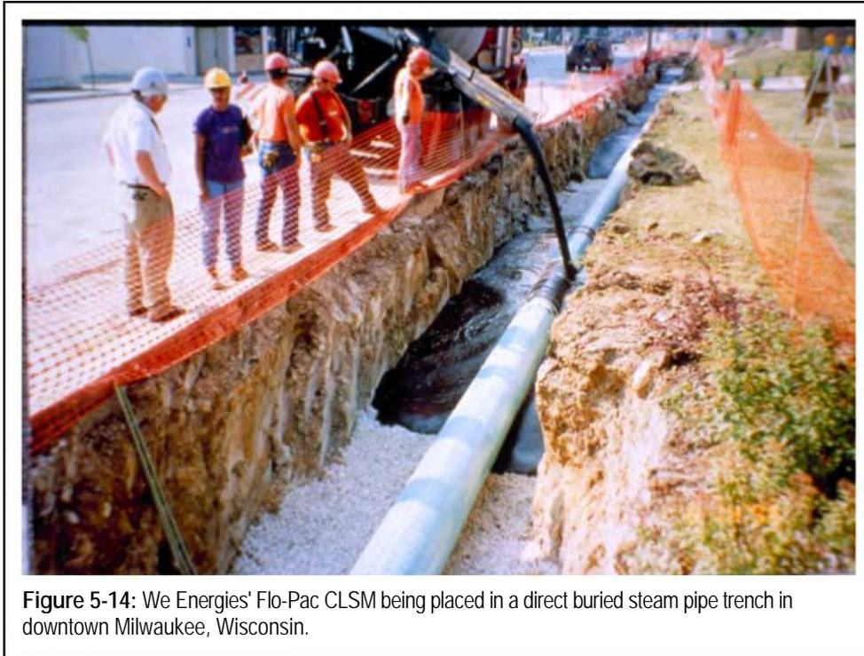
Figure 5-14: We Energies' Flo-Pac CLSM being placed in a direct buried steam pipe trench in downtown Milwaukee, Wisconsin.
