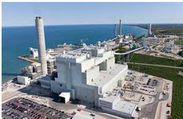
This 1,230 MW pulverized coal-fueled plant is located along the shore of Lake Michigan near the existing Oak Creek Power Plant (OCP). The OCXP was formerly known as Elm Road Generating Station (ERGS). Based on current projections, it is estimated that by burning eastern bituminous coal, it will
