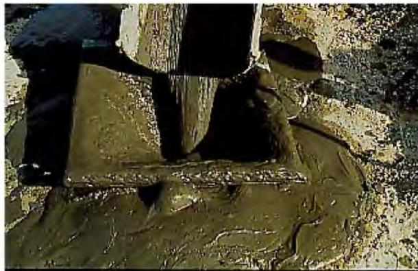
Figure 5-13: CLSM flowing through a funnel to fill an underground tunnel in downtown Milwaukee, Wisconsin.
