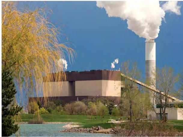
This 1,210 MW, pulverized coal-fueled plant is located in the town of Pleasant Prairie in Kenosha County. Each year the plant produces approximately 225,000 tons of fly ash, 53,000 tons of bottom ash and 76,000 tons of FGD gypsum by burning a blend of low sulfur western sub-bituminous coals from the Wyoming Powder River
