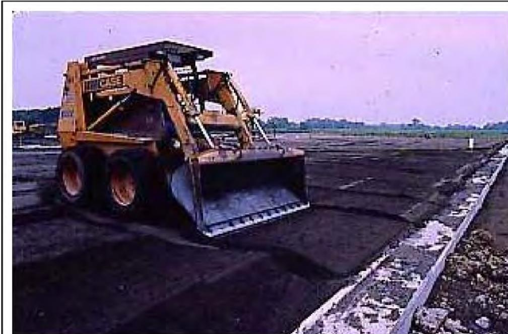
Figure 6-4: Bottom ash structural backfill being used for building construction in Racine, Wisconsin
