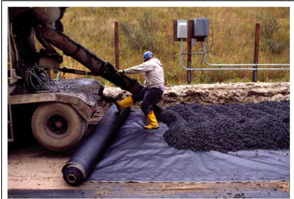
Figure 4-26: Open-graded cementitious base course material being placed over filter fabric at Port Washington Power Plant's high-volume fly ash concrete pavement demonstration project.
