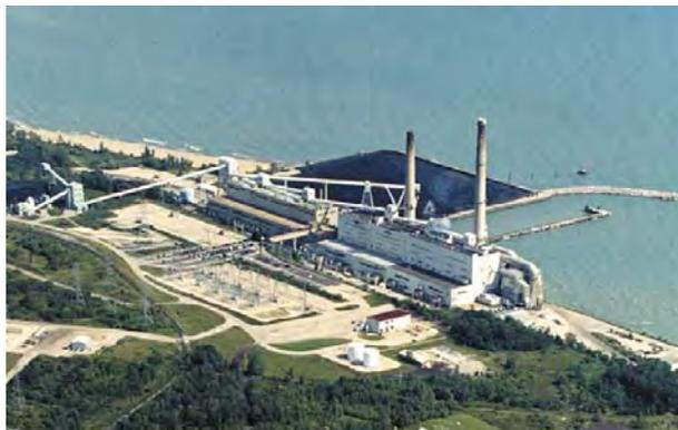
This 1,135 MW pulverized coal-fired plant is located in the city of Oak Creek, Milwaukee County, near the Milwaukee-Racine county line. It supplies electrical energy to the company's power grid and produced approximately 99,000 tons of fly ash, 22,000 tons of bottom ash,
