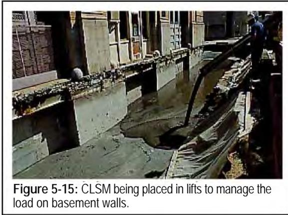
Figure 5-15: CLSM being placed in lifts to manage the load on basement walls.
