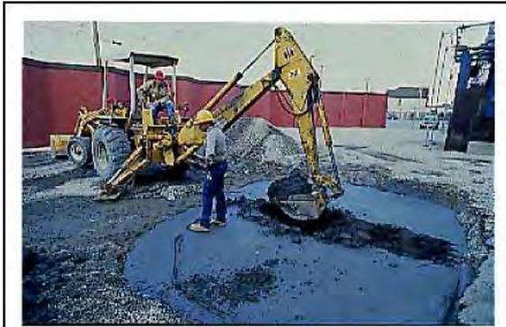
**Figure 5-9:** Excavating hardened CLSM with a backhoe at We Energies Valley Power Plant in downtown Milwaukee, Wisconsin.
