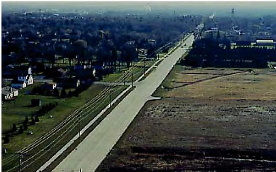
Figure 4-20 : Maple Avenue roadway and sidewalk located in the village of Sussex and paved with high-volume fly ash concrete.
