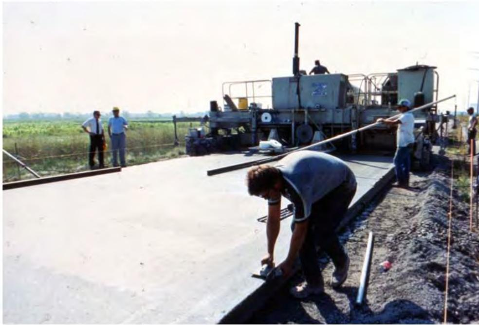
**Figure 4-22:** Finishing touch to We Energies' high-volume fly ash concrete demonstration project at Pleasant Prairie Power Plant.
