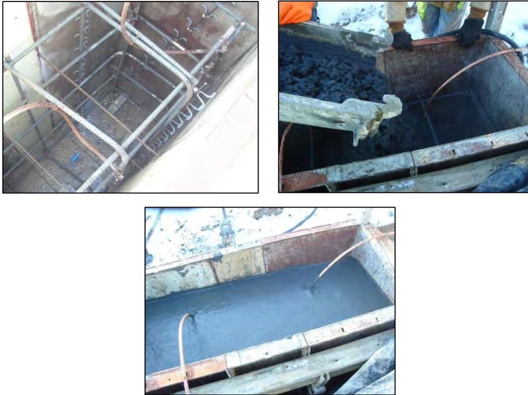
Figure 4-34: The placement of conductive concrete slab during construction at the Caledonia Landfill site
