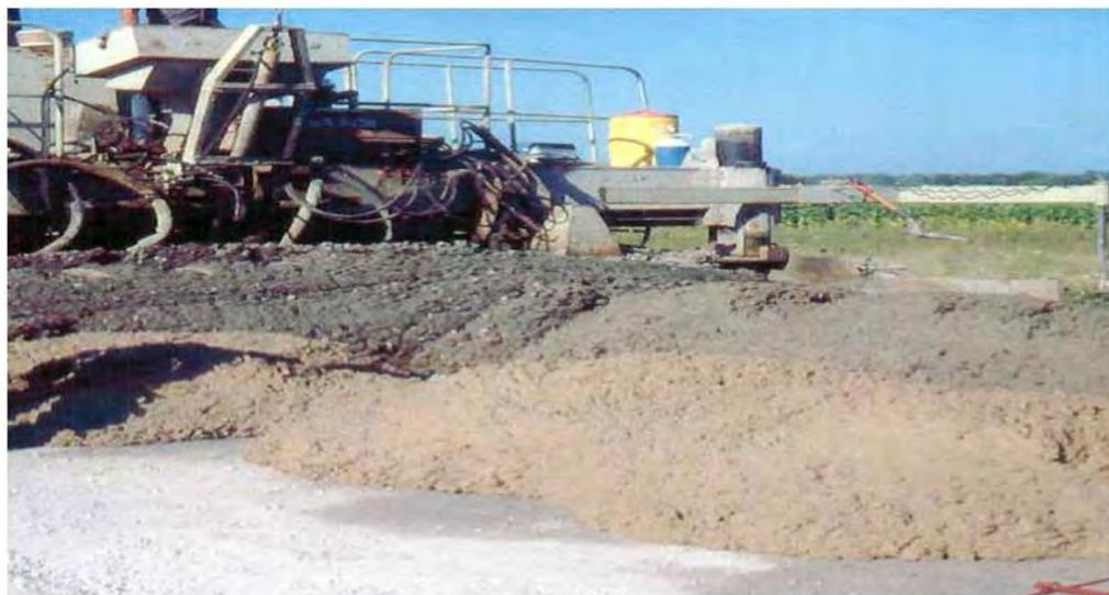
**Figure 4-23:** High-volume fly ash demonstration road paving at Pleasant Prairie Power Plant. Note the difference between the darker slate colored class F fly ash concrete and lighter tan colored high-volume class C fly ash concrete.
