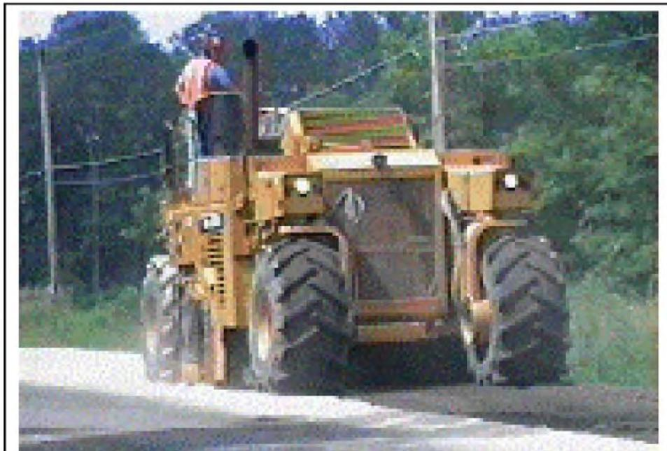
Figure 8-2: Pavement being repulverized after fly ash application.
