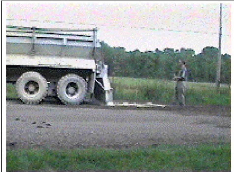
Figure 8-1: Fly ash being placed uniformly on the pulverized pavement.
