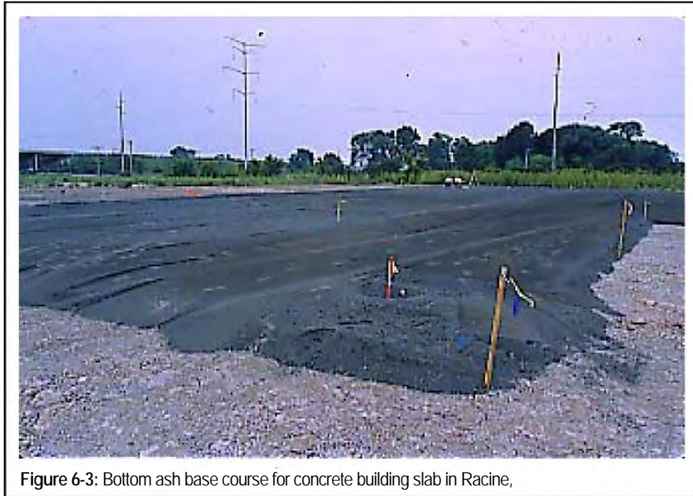
Figure 6-3: Bottom ash base course for concrete building slab in Racine,
