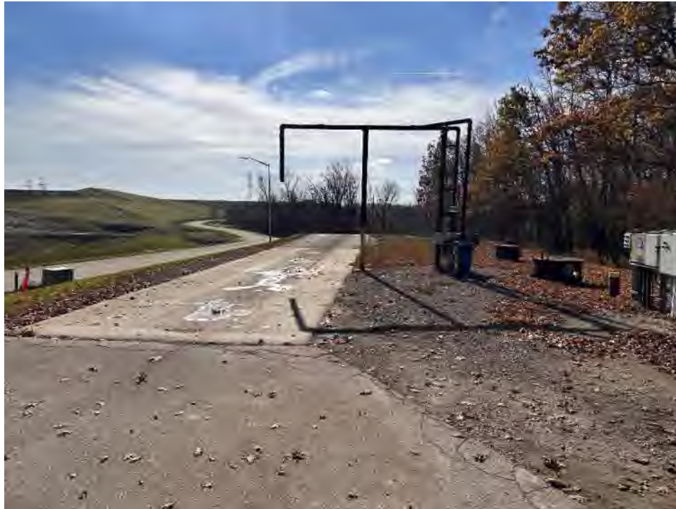
Photo No. 9 – Leachate load-out facility.
