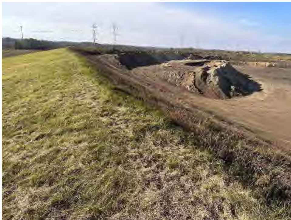
Photo No. 2 – Stockpiled CCR inside Cell 2.
