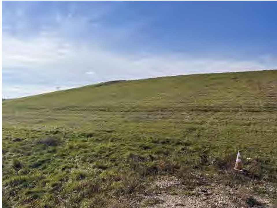
Photo No. 7 – Vegetation on Cell 6 and 8 perimeter slope.
