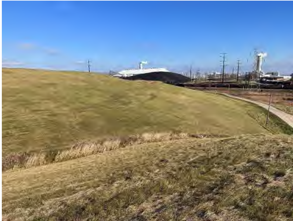
Photo No. 5 – South perimeter berm looking northeast.
