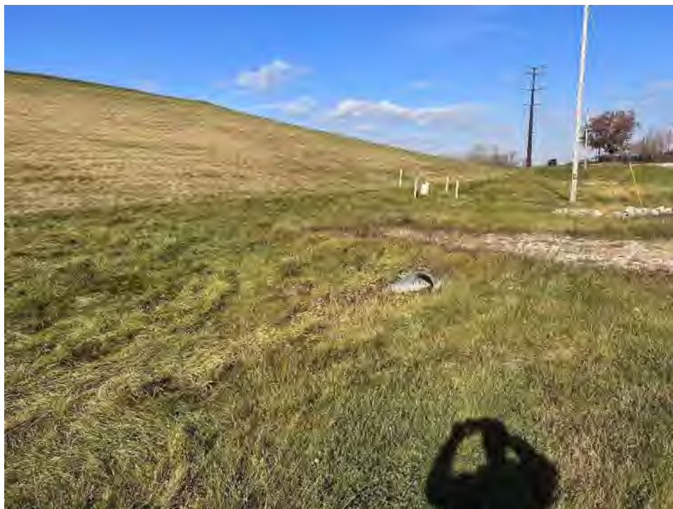
Photo No. 6 – East perimeter berm and stormwater ditch, looking north.
