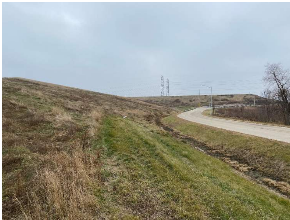
Photo No. 4: West perimeter berm looking south 12/07/2022
