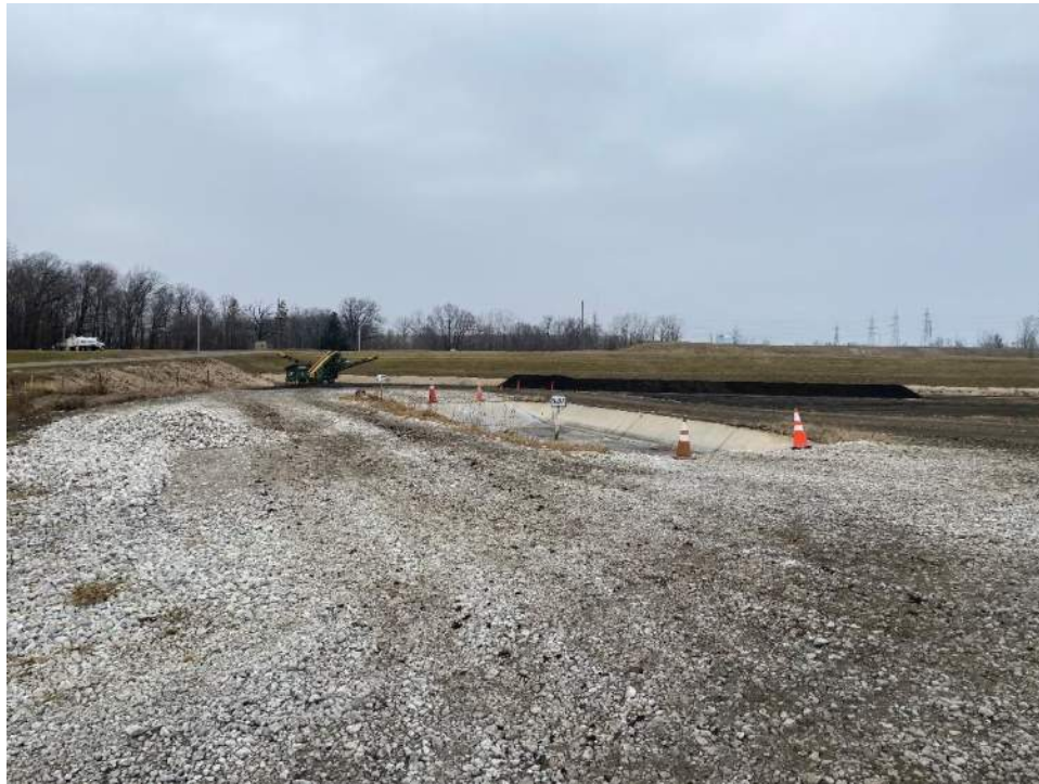
Photo No. 3: Tire wash in Cell 8 looking north on 12/07/2022
