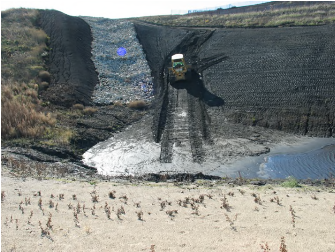
Repairing Erosion in East Stormwater Storage Area
