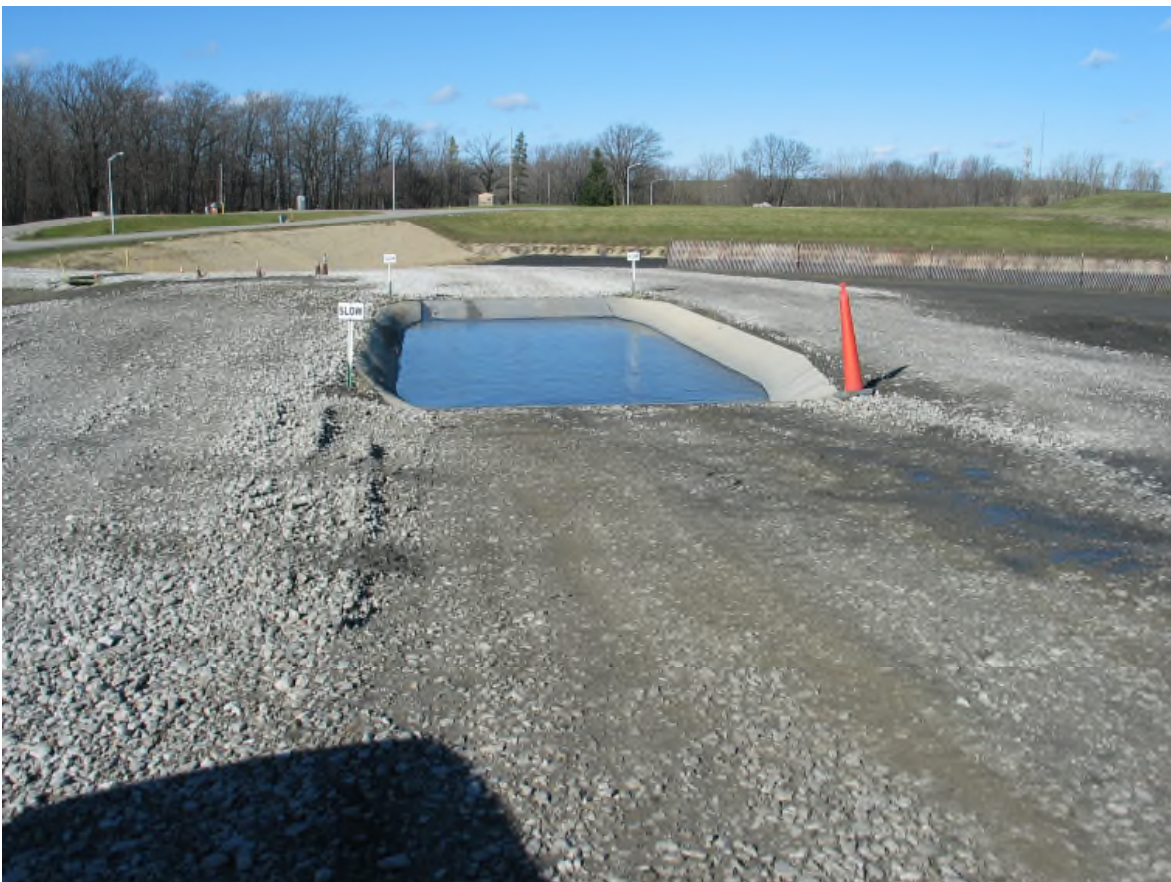
Wheel Wash at Cell Entrance/Exit
