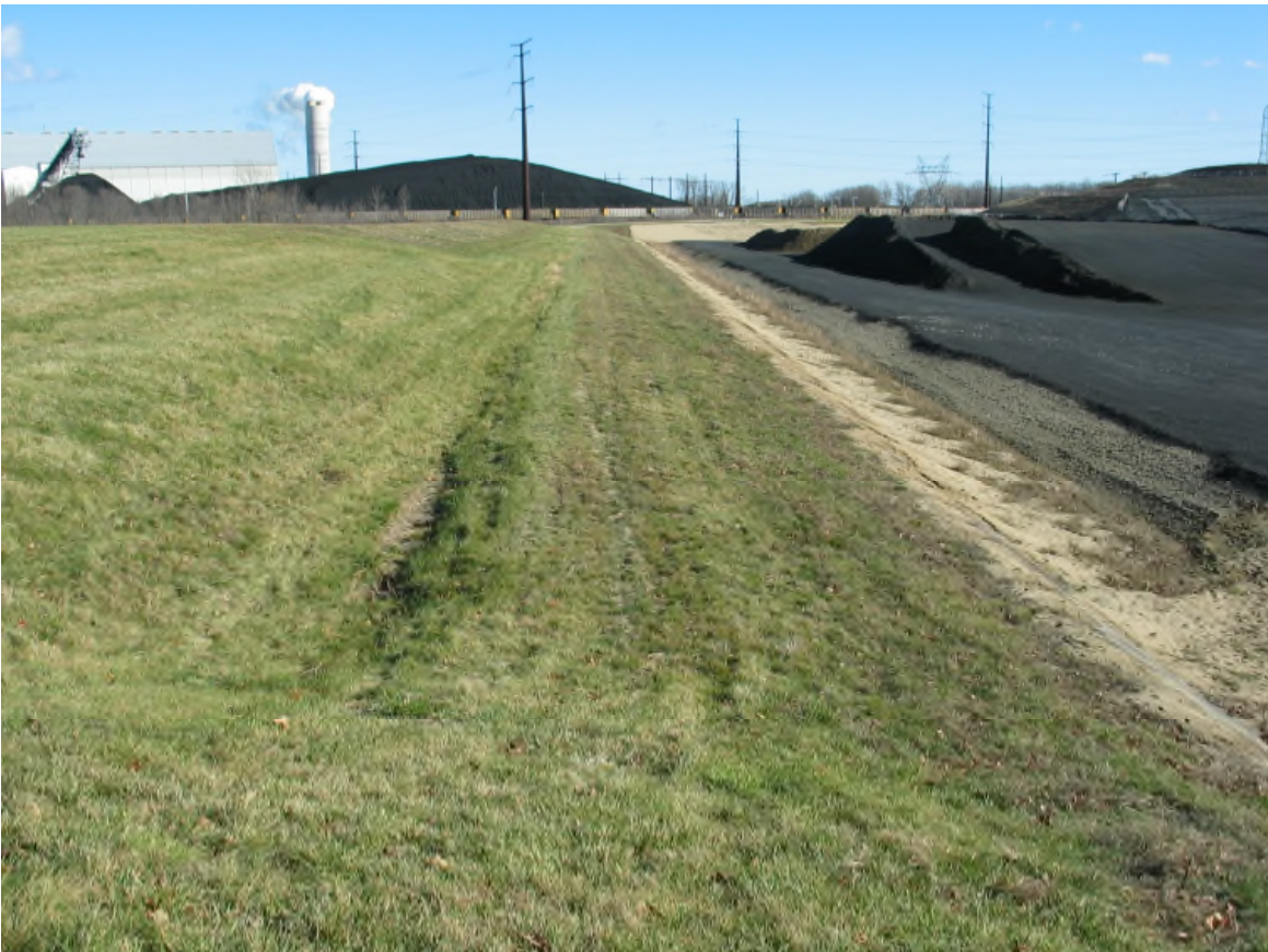
North Perimeter (Intercell) Berm (looking east)
