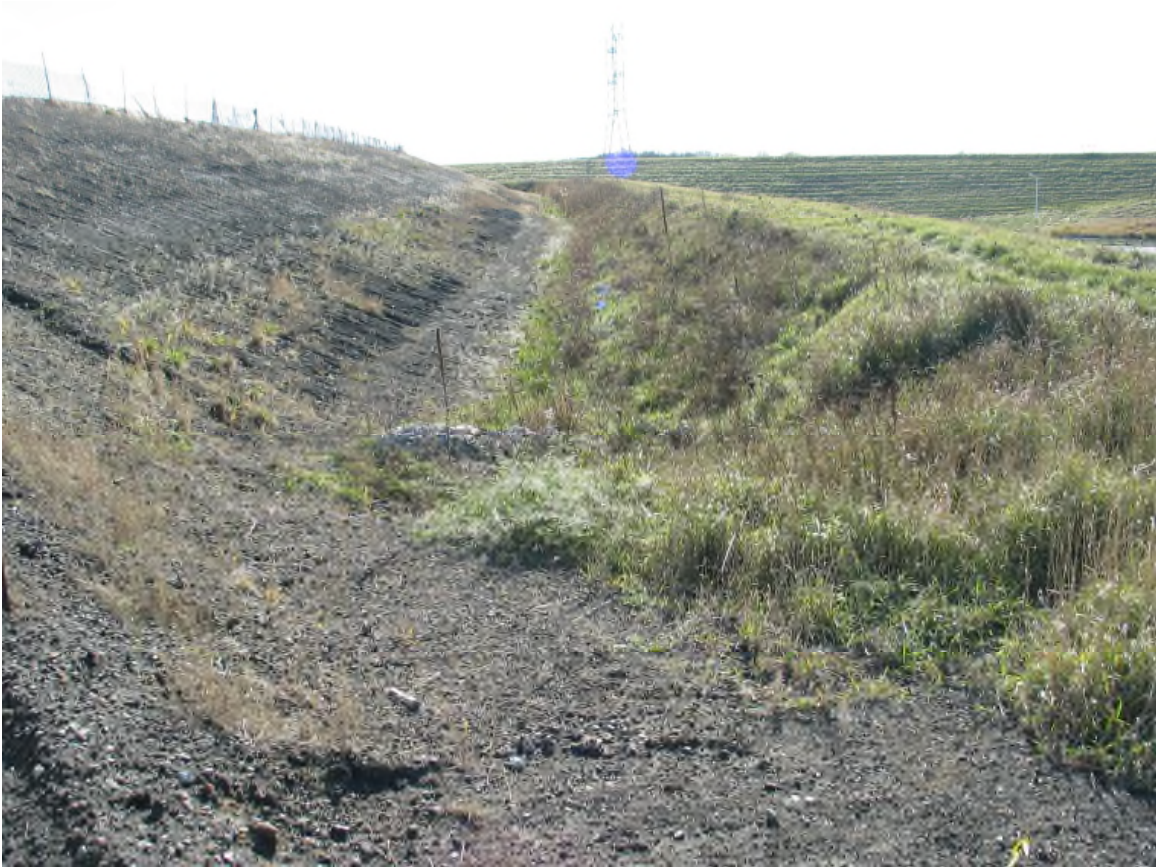
West Perimeter Upper Berm (looking south)
