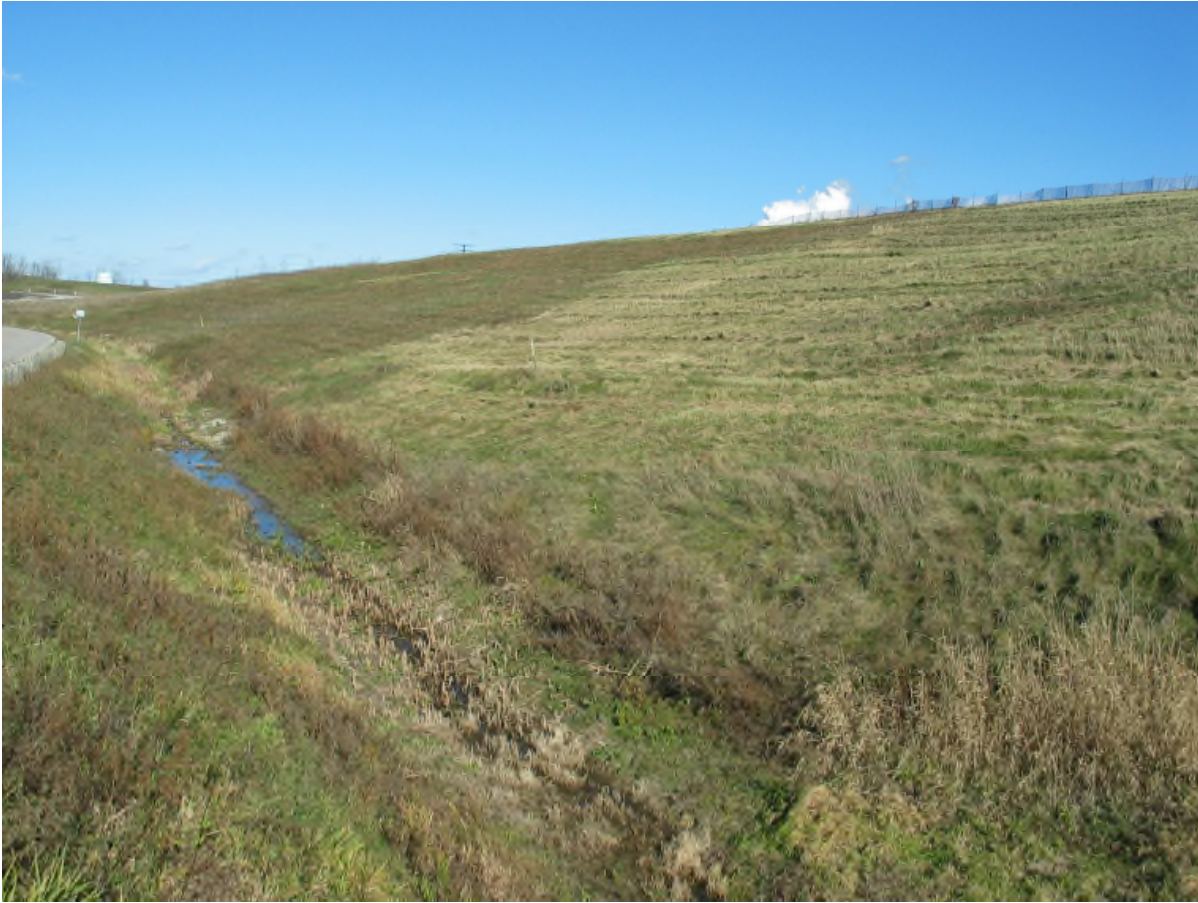
West Side Final Covers (looking north)
