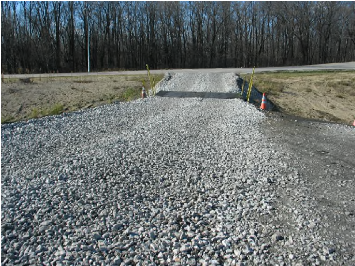
Cell Entrance (looking west)
