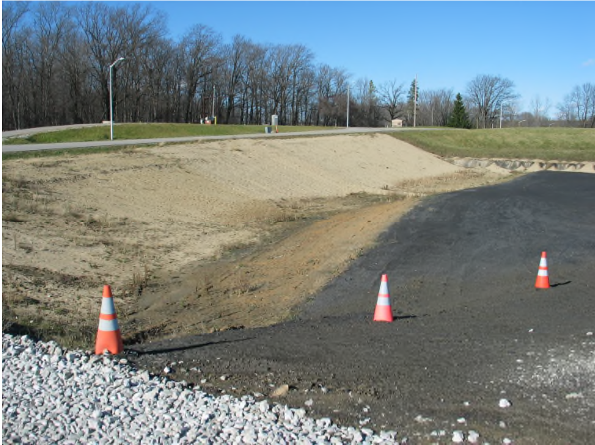
West Berm Cell 10 (looking north)
