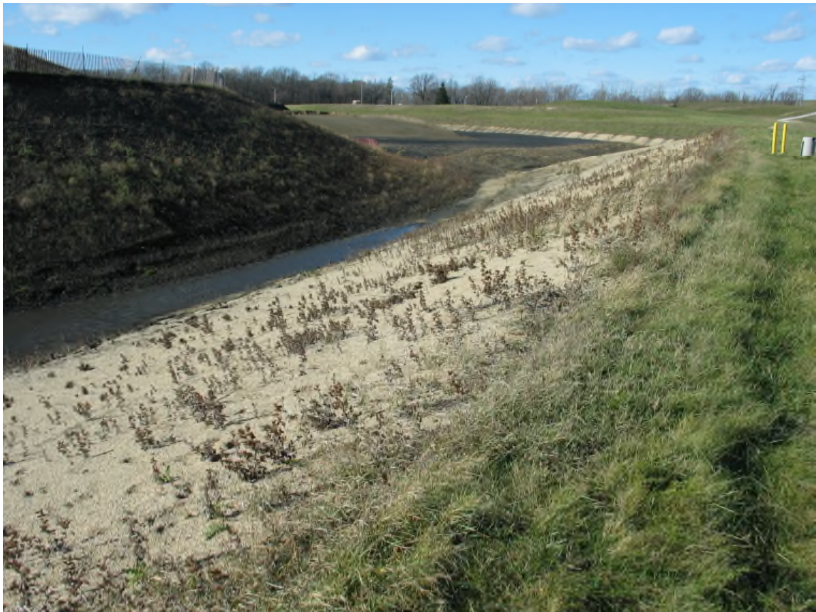
East Perimeter Berm (looking north)
