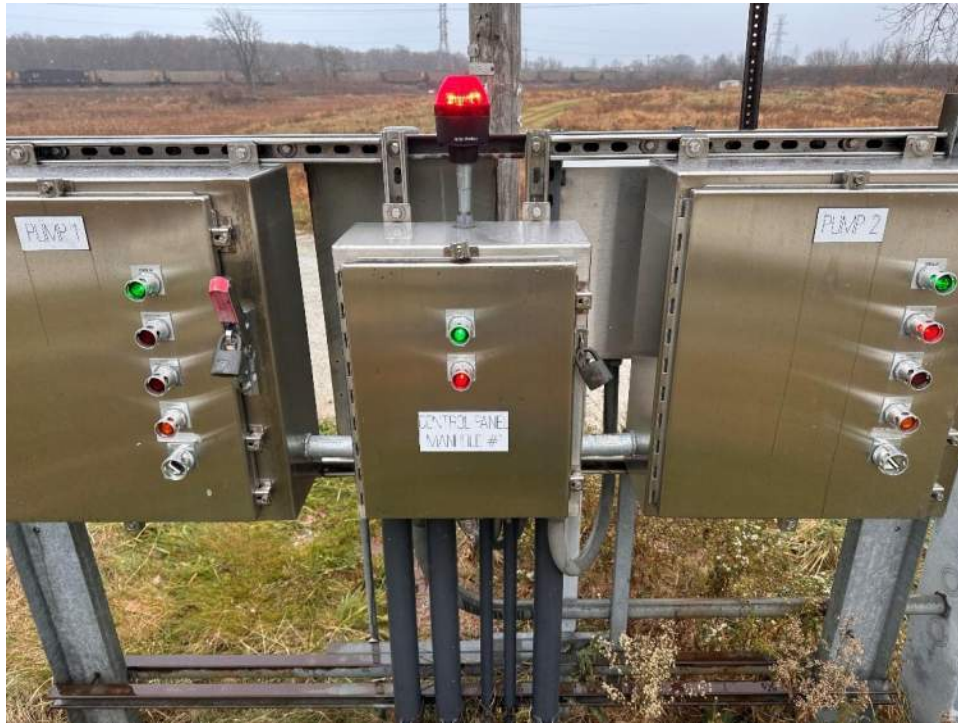
Photo No. 9 – Leachate tank control panel.
