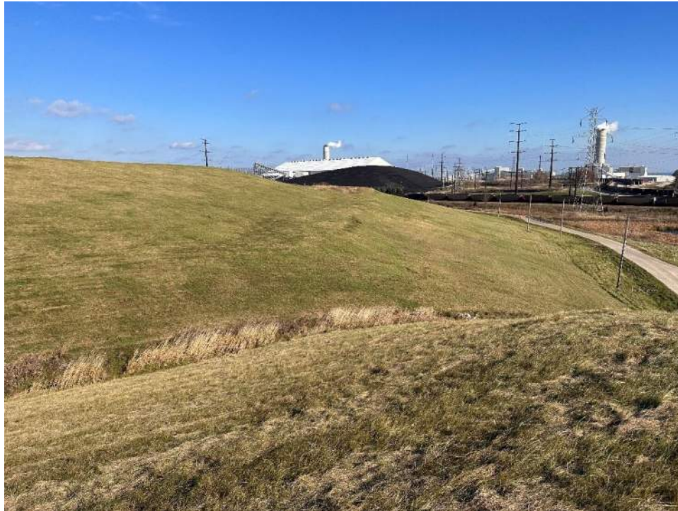
Photo No. 5 – South perimeter berm looking northeast.
