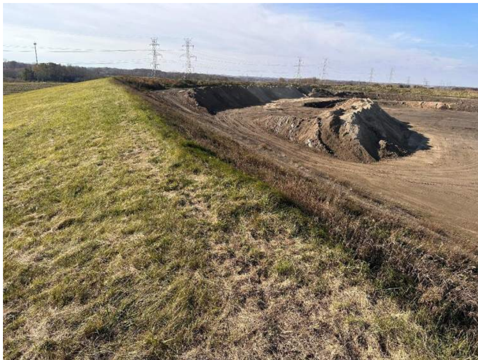
Photo No. 2 – Stockpiled CCR inside Cell 2.
