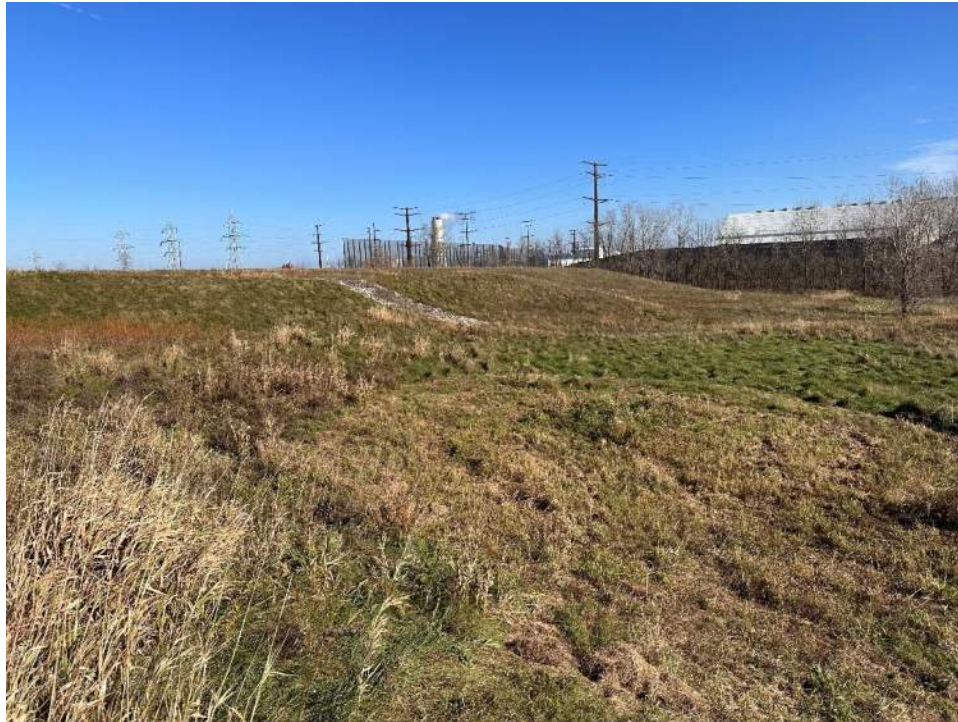
Photo No. 11 – Fully vegetated cover soil stockpile located north of the landfill.
