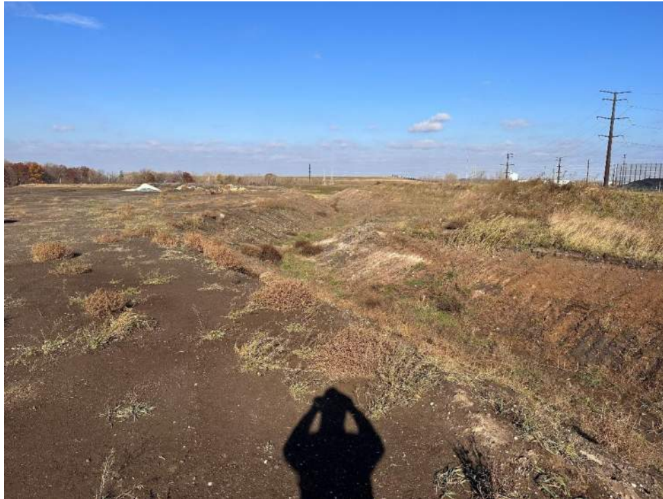
Photo No. 3 – Leachate collection ditch behind Cell 6 and 8 partial cover.
