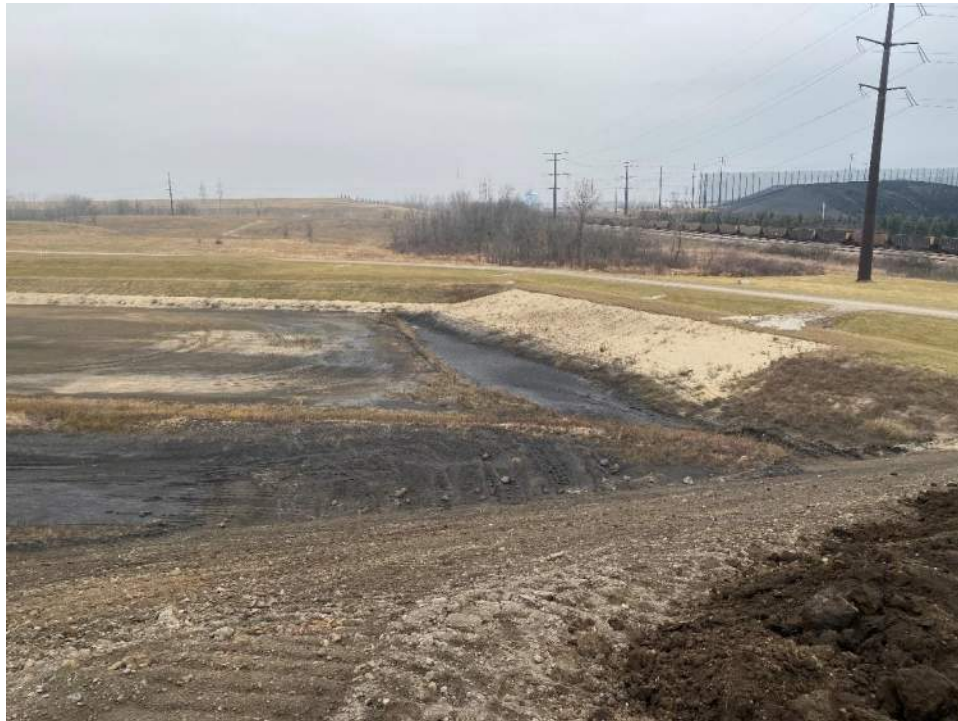
Photo No. 1: East interior berm of Cell 10 looking north 12/07/2022
