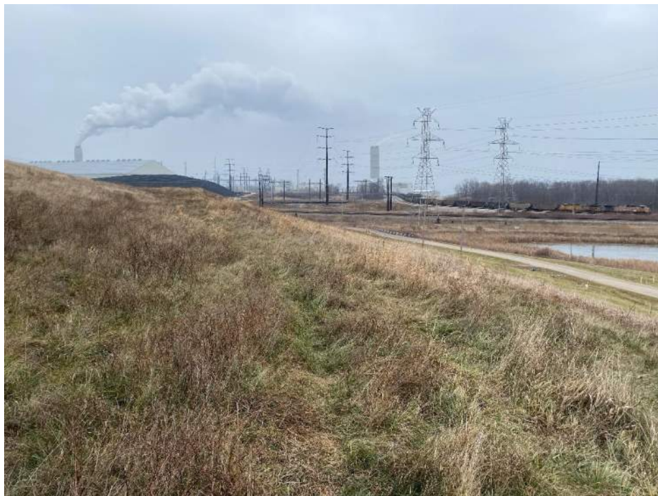
Photo No. 6: South perimeter berm looking east on 12/07/2022
