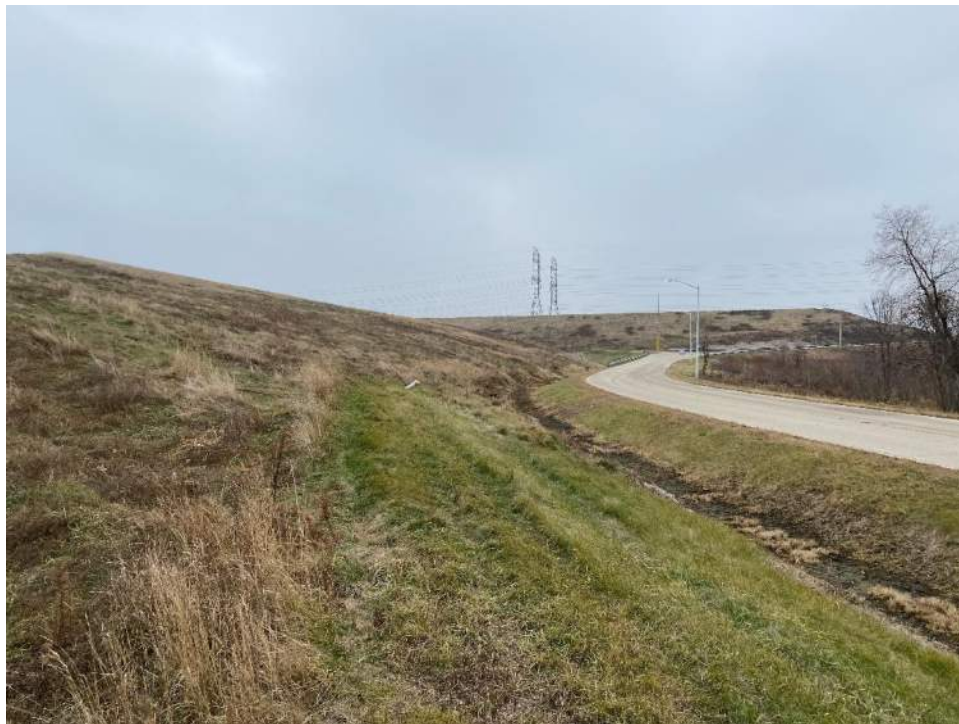
Photo No. 4: West perimeter berm looking south 12/07/2022
