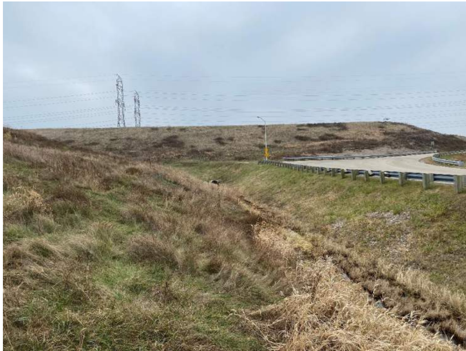
Photo No. 5: West perimeter berm looking south 12/07/2022
