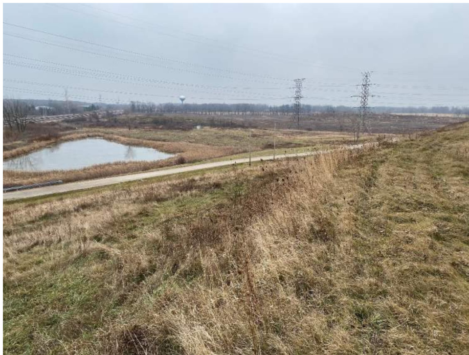
Photo No. 8: East perimeter berm looking south 12/07/2022
