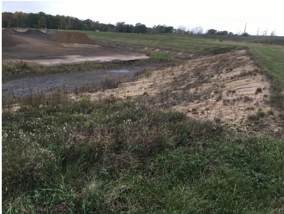
Photo No. 3: East perimeter berm looking north 10/12/2021
