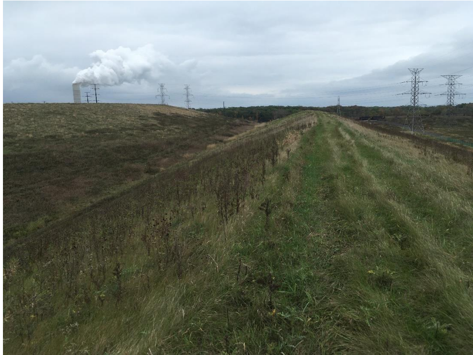
Photo No. 9: South slope of the Caledonia Landfill looking east 10/12/2021
