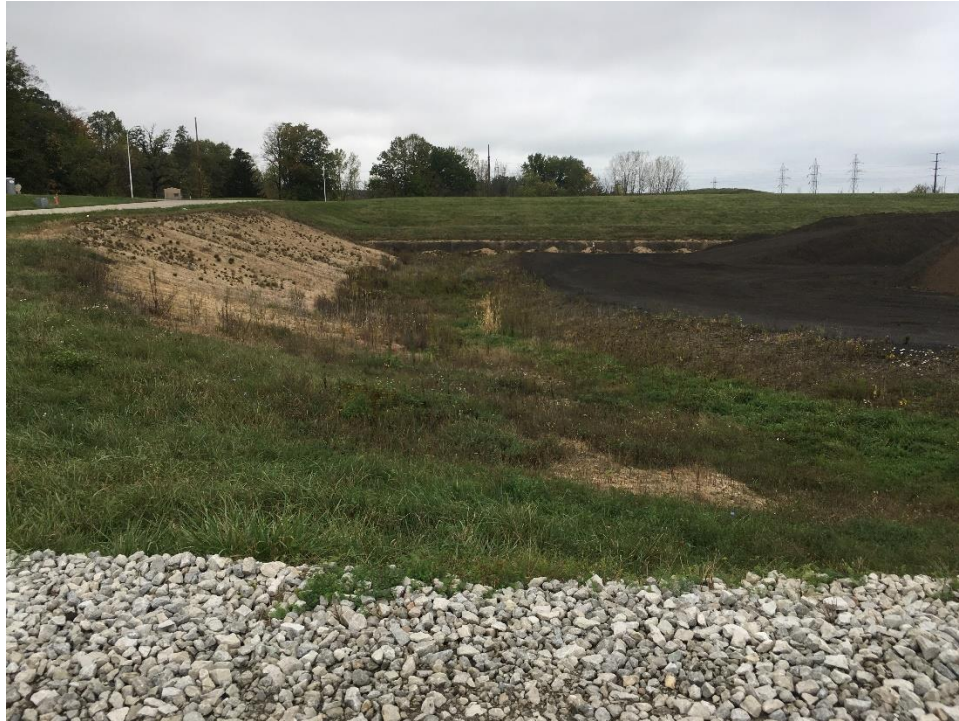
Photo No. 5: West interior slope of Cell 10 looking north on 10/12/2021
