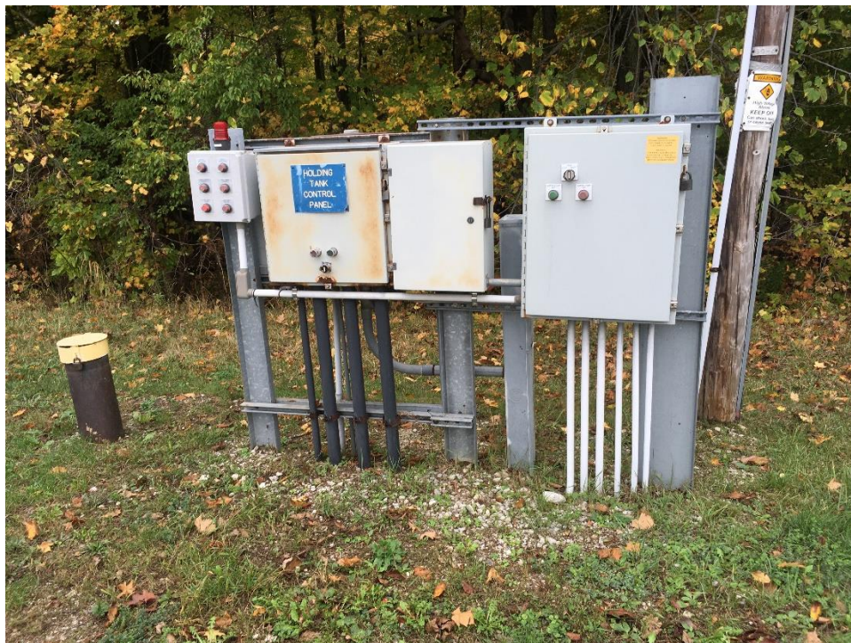
Photo No. 12: Holding tank control panel for leachate loadout facility 10/12/2021
