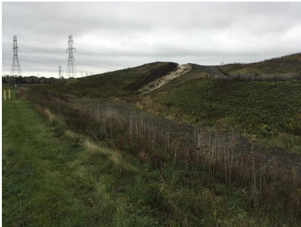
Photo No. 4: East perimeter berm looking south 10/12/2021
