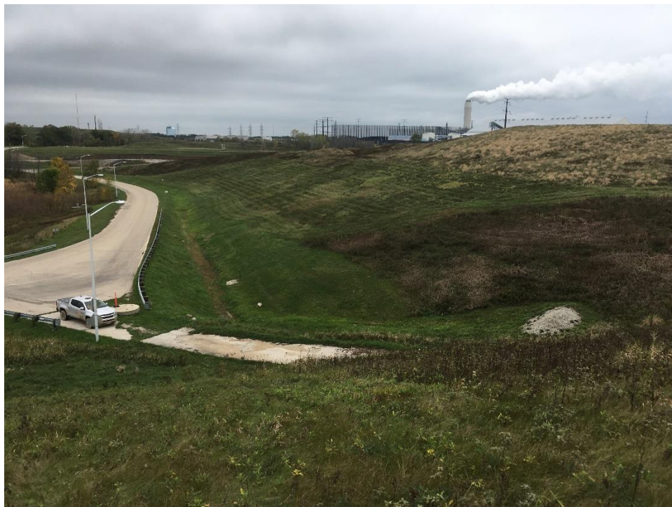
Photo No. 8: West perimeter slope looking north 10/12/2021
