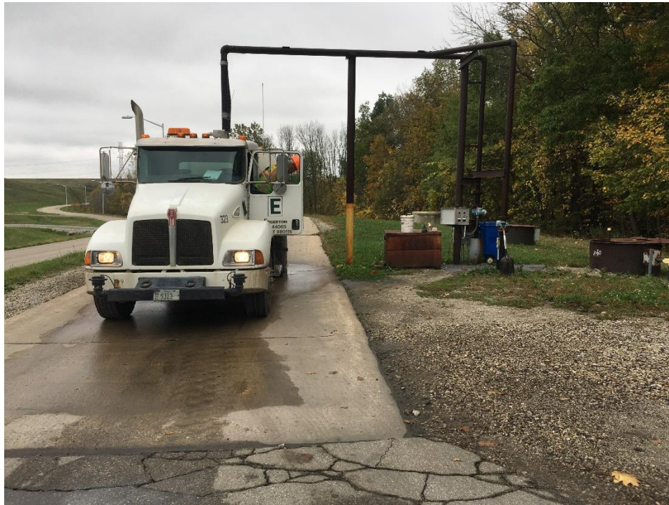
Photo No. 11: Leachate loadout facility looking south 10/12/2021
