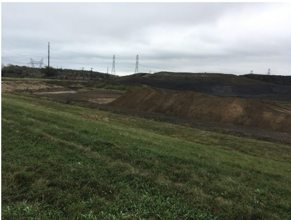
Photo No. 2: North perimeter limit of Cell 10 looking southeast on 10/12/2021
