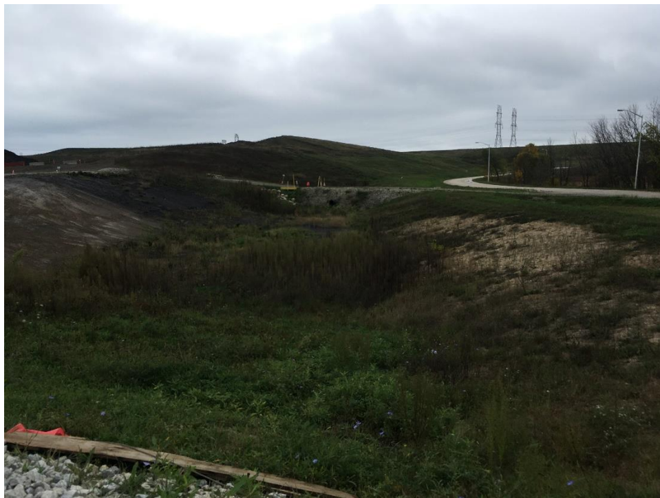
Photo No. 6: West interior slope looking south 10/12/2021
