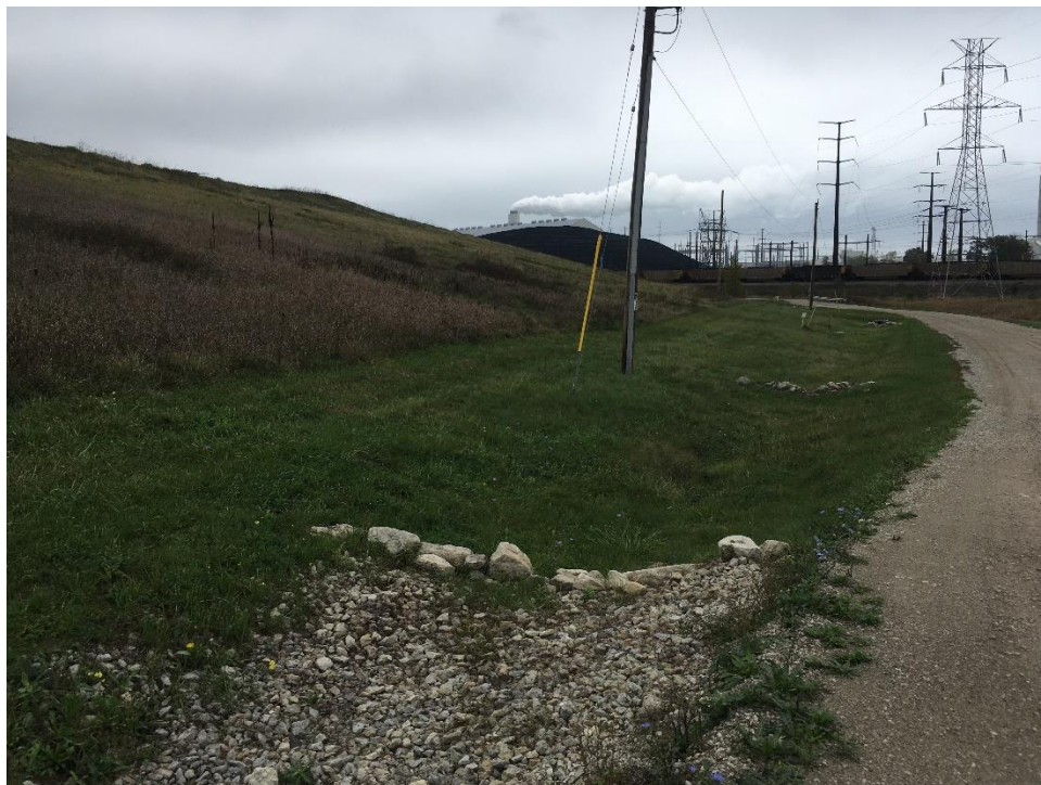
Photo No. 10: East slope of the Caledonia Landfill looking north-northeast 10/12/2021
