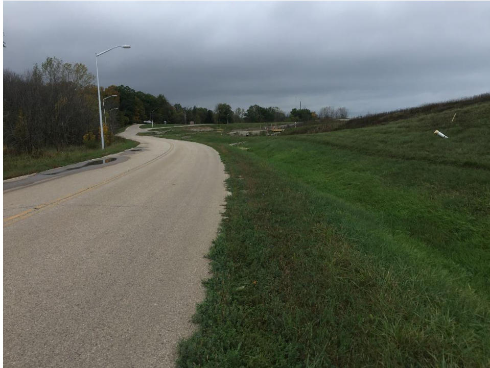
Photo No. 7: West perimeter slope and stormwater ditch looking north 10/12/2021
