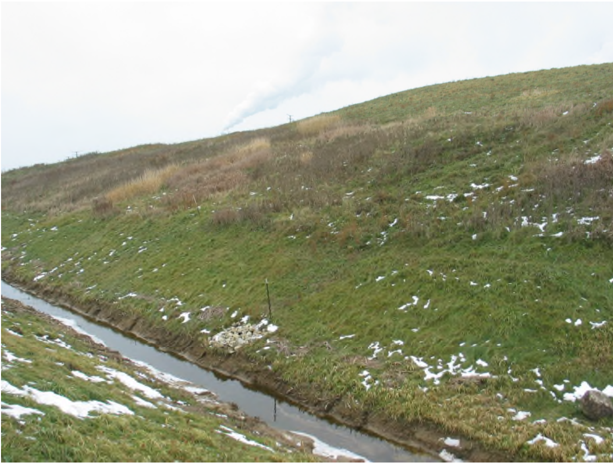
Final cover & perimeter ditch (west side)
