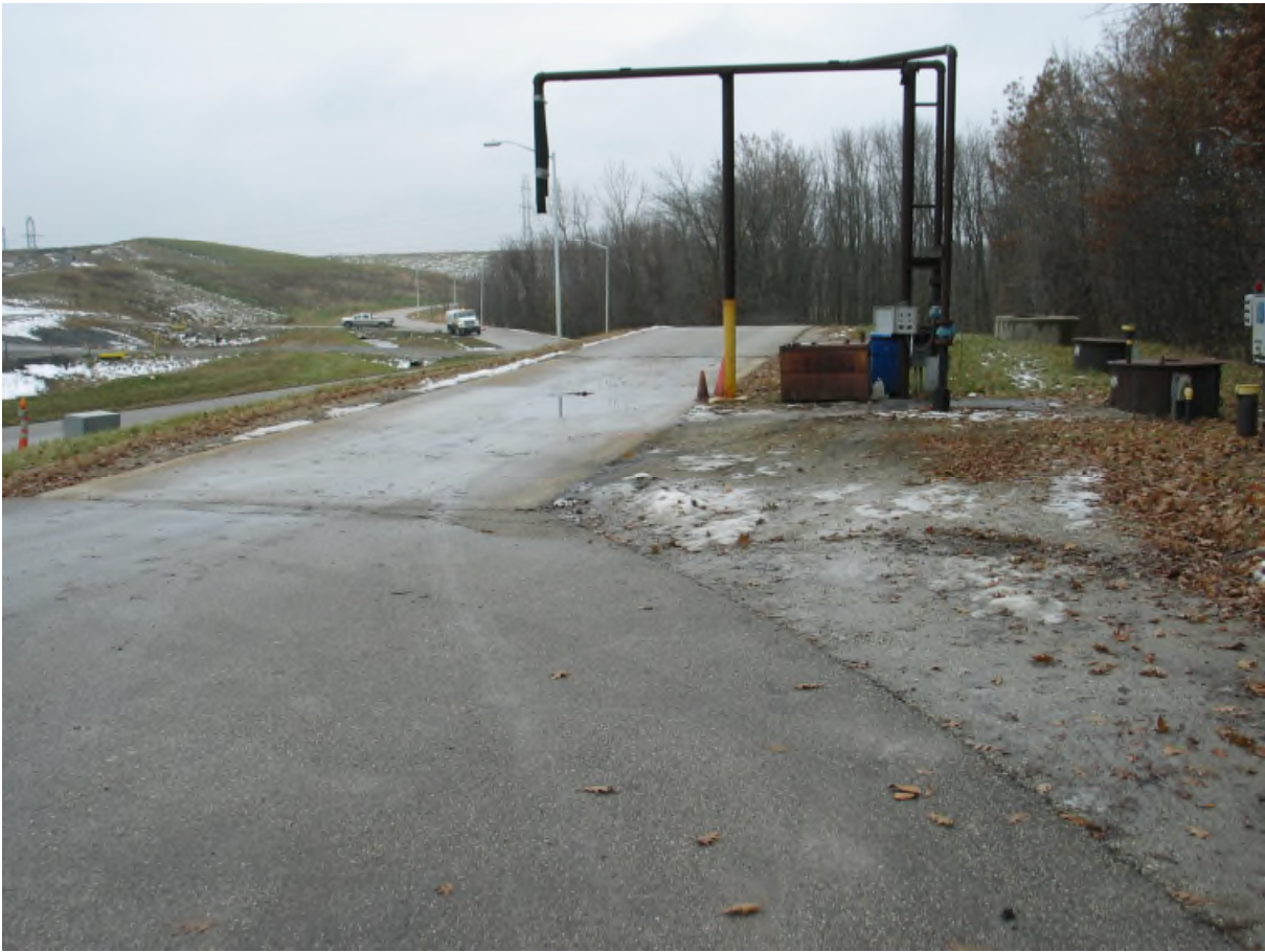
Leachate load-out (looking south)
