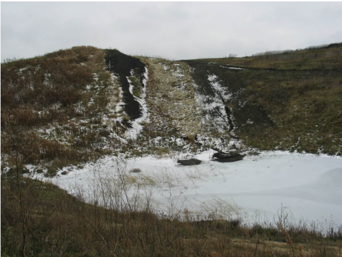
Upper area letdown flume (looking south)
