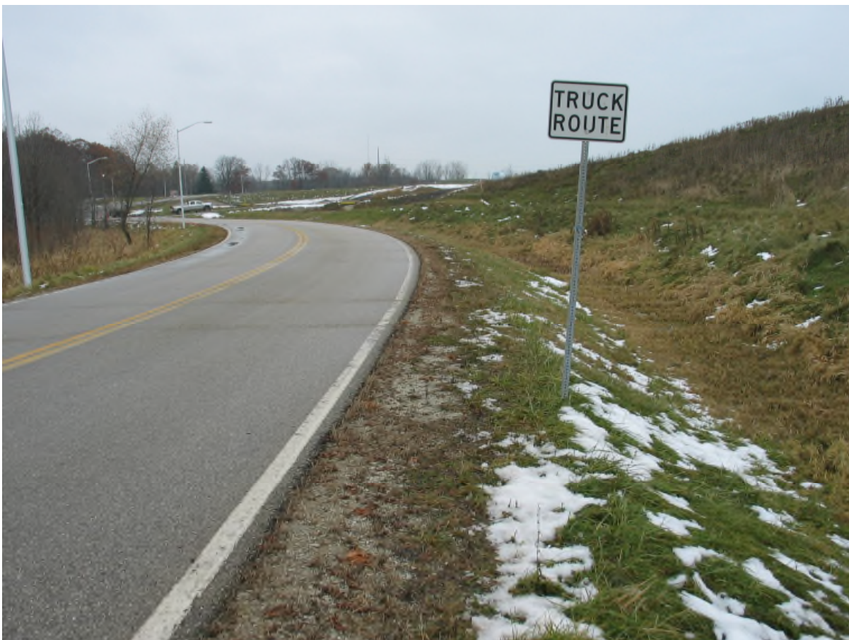
Access Road (looking north)
