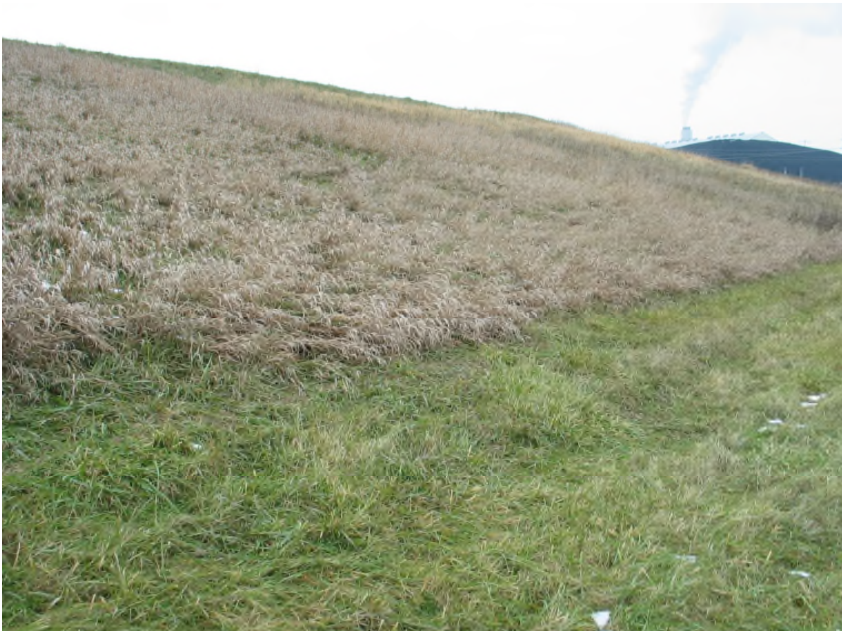
East side final cover (looking northeast)
