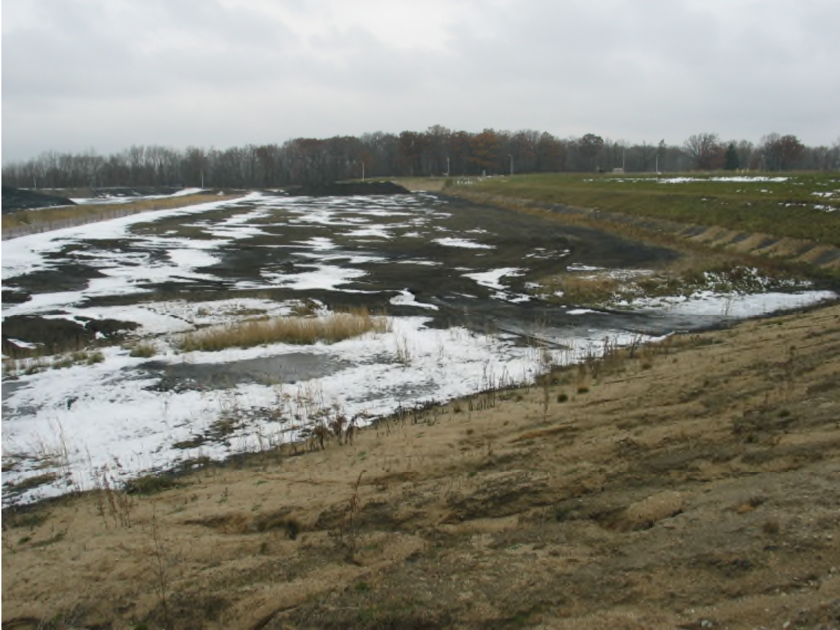
Bottom ash storage area Cell 10 (looking west)
