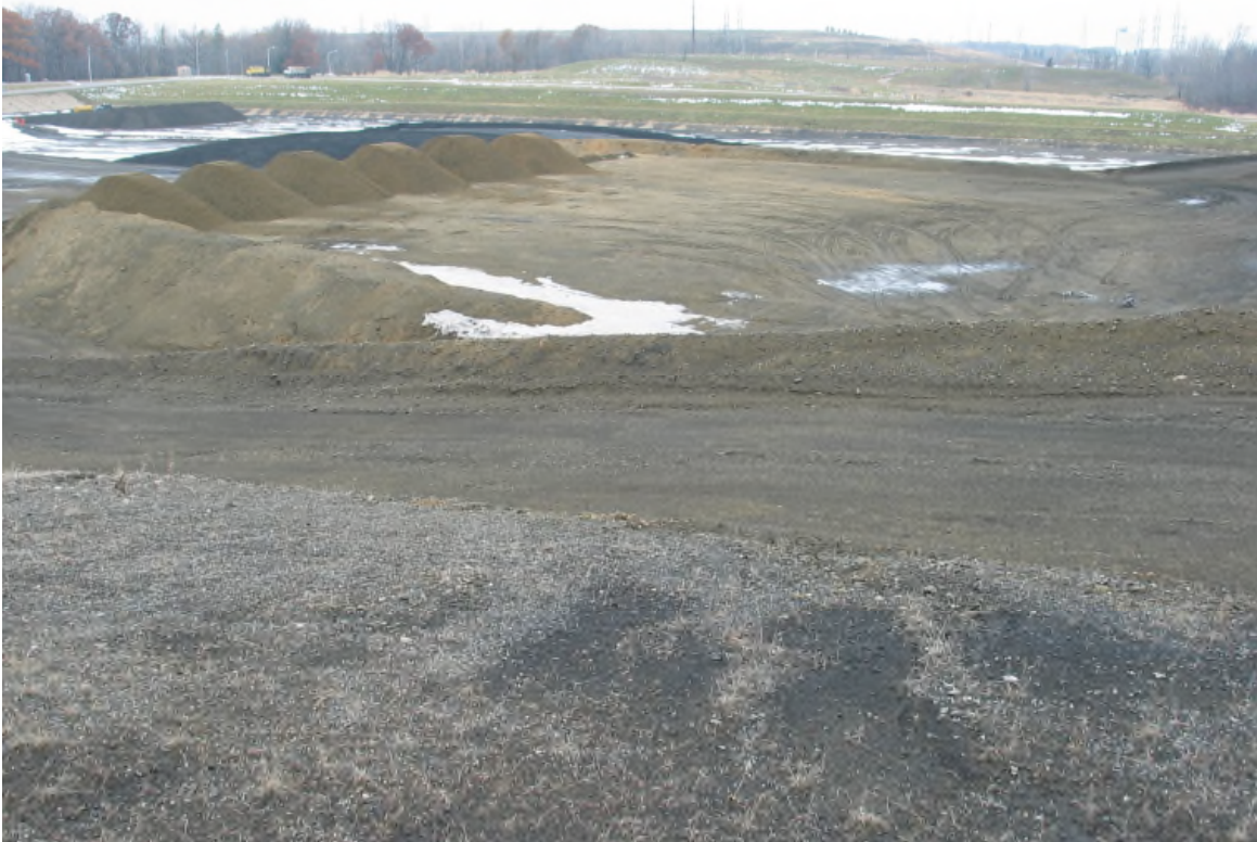
OCPP bottom ash storage area Cell 8 (looking north)
