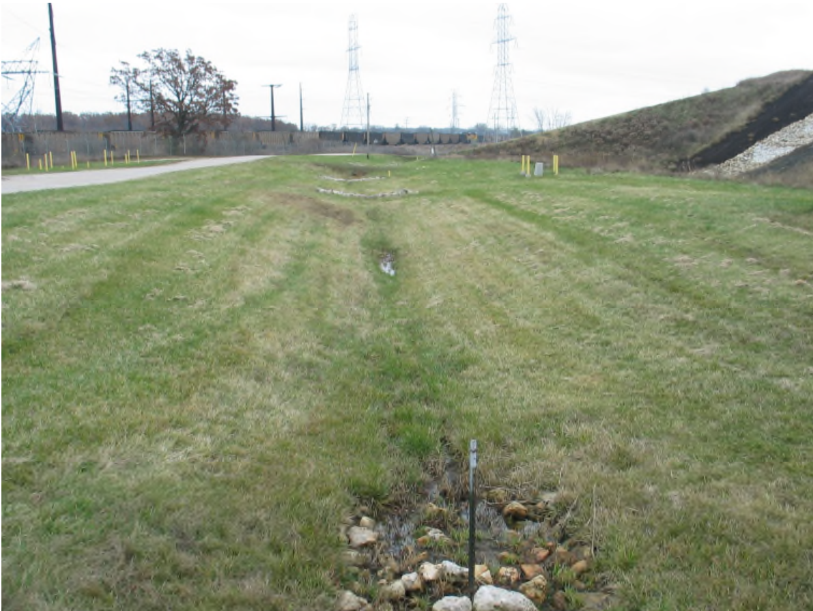
East Side Surface Water Ditch (looking south)
