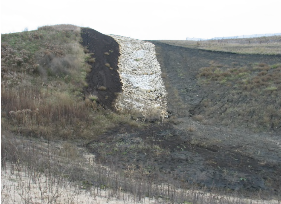
Down Flume from Upper Cells (looking southwest)
