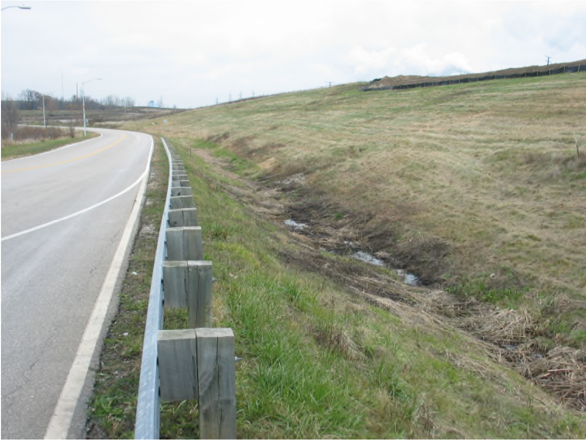
West Side Final Covers & Surface Water Ditch (looking north)
