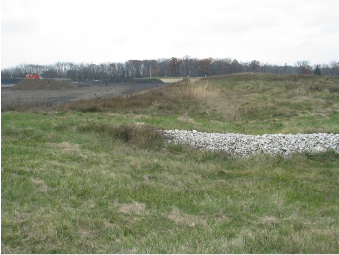
North Intercell Berm (looking west)
