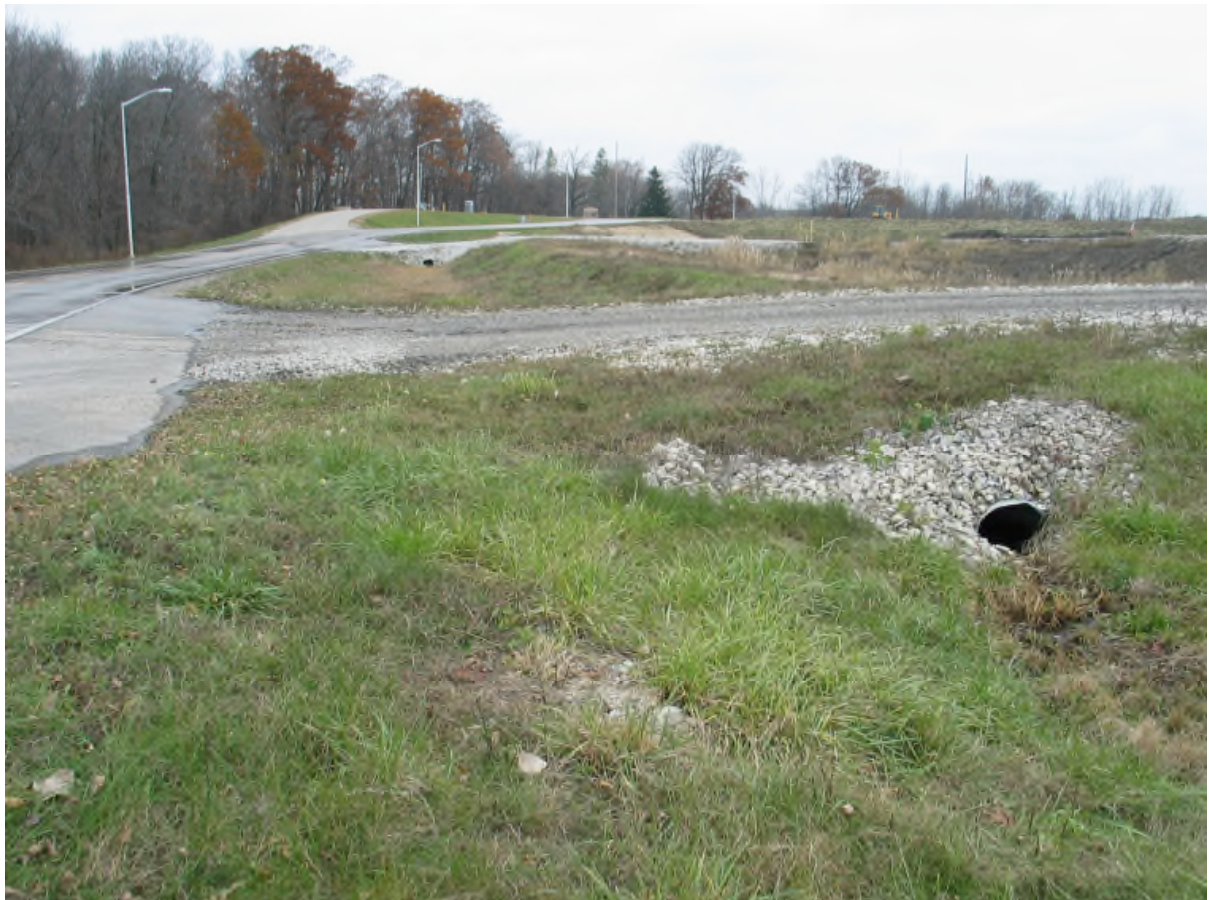
West Berm (looking north)
