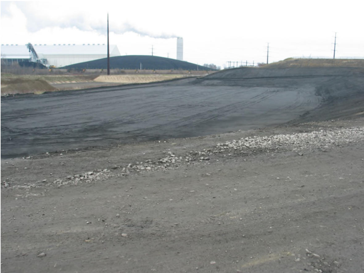
Groomed Waste Surface Cell 8 (looking east)
