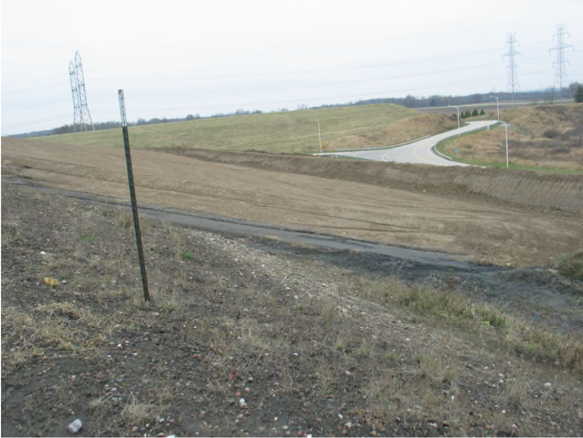
Northwest End Upper Cells & New Cover Construction (looking south)
