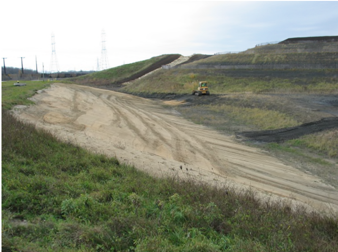
East Perimeter Berm (looking south)
