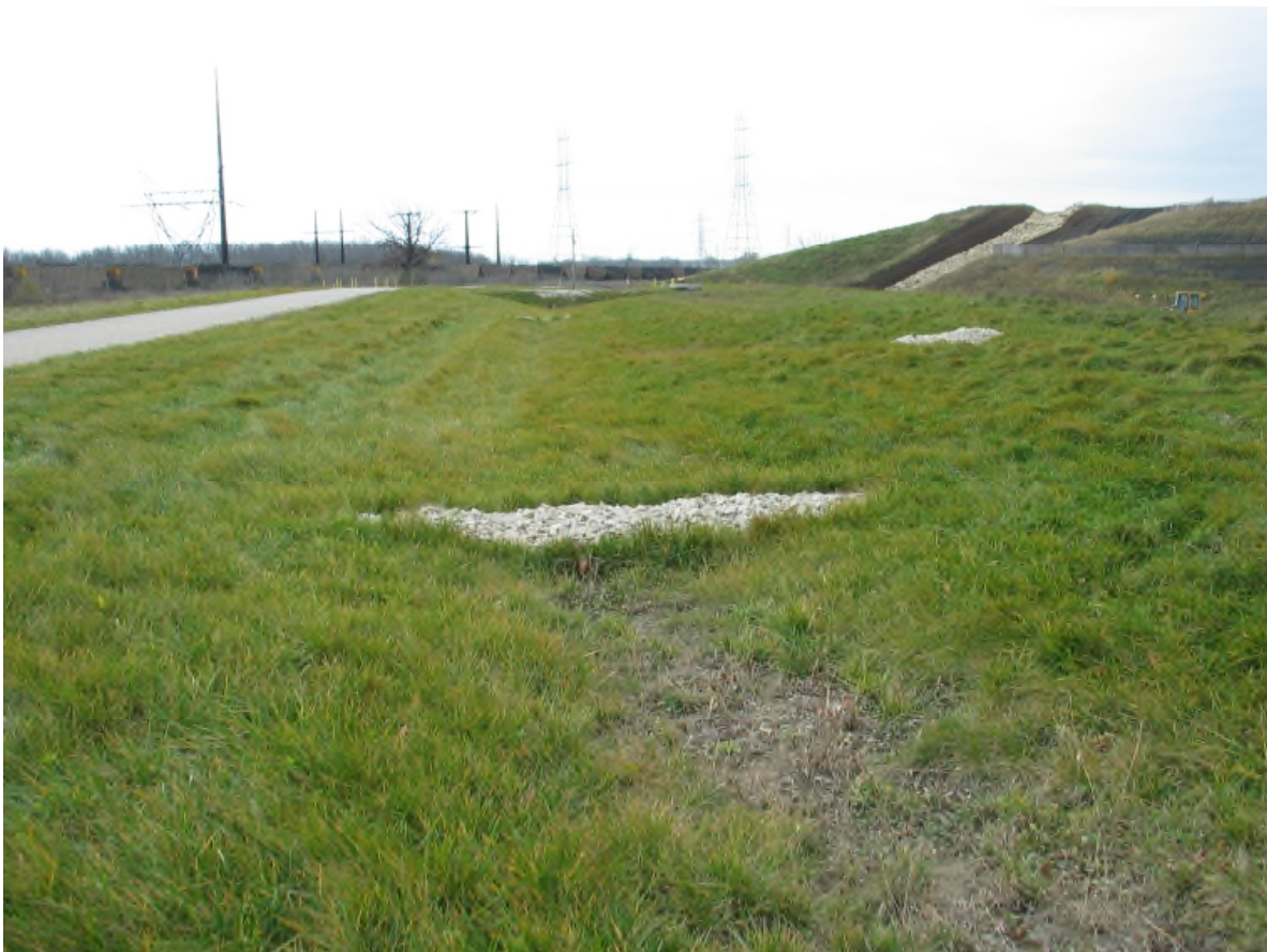
East Side Surface Water Ditch (looking south)
