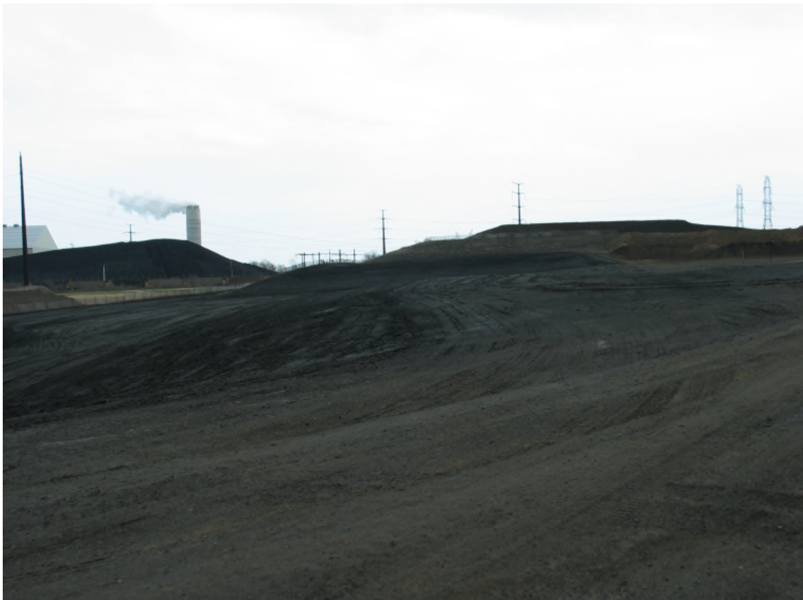
Groomed Waste Surface Cell 8 (looking east)
