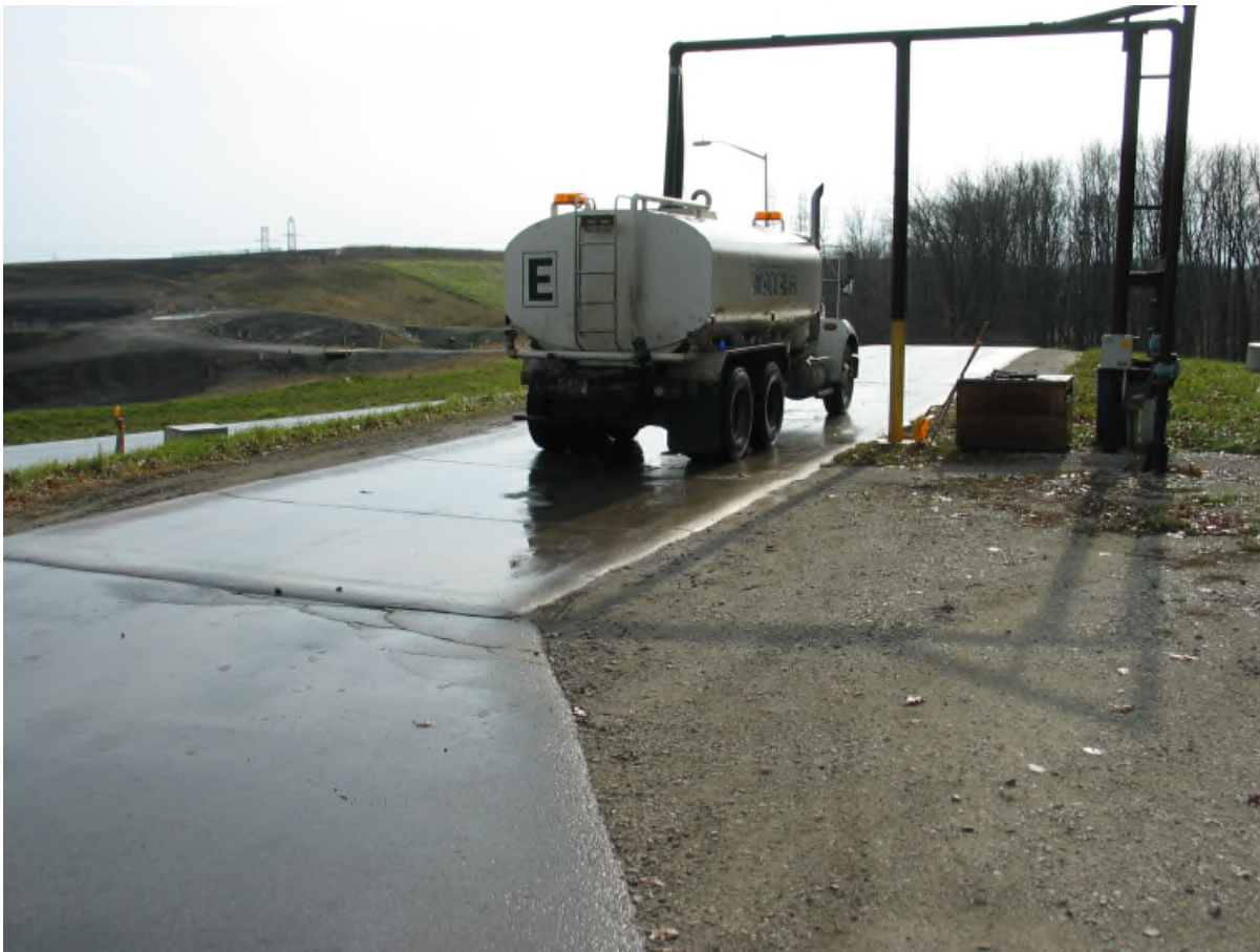
Leachate Load-Out (looking south)
