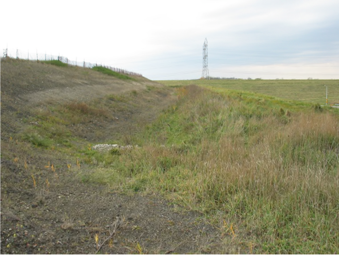
Northwest End Upper Run-off Control Ditch (looking south)
