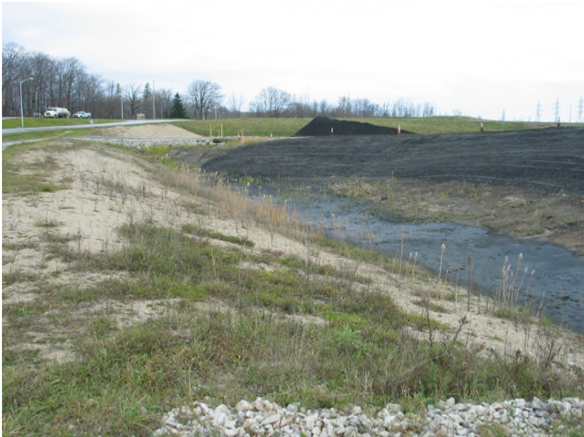
West Berm (looking north)
