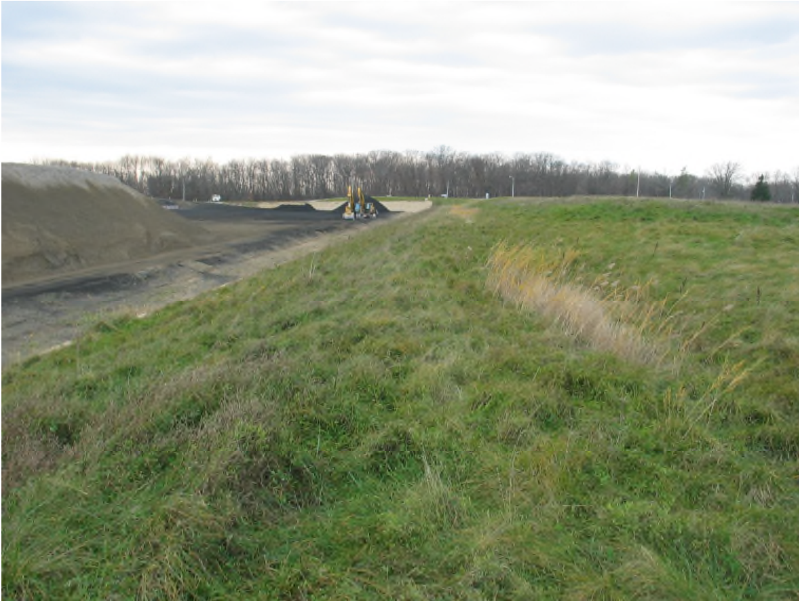
North Intercell Berm (looking west)
