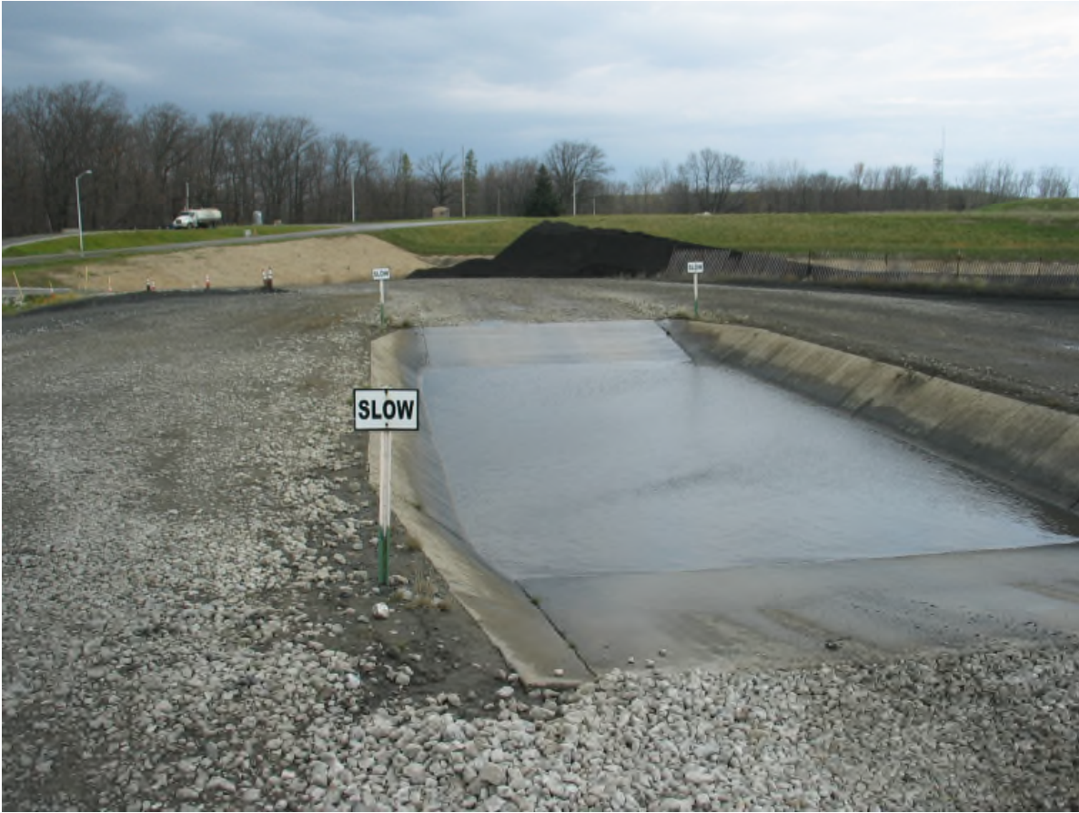
Tire Wash (looking north)
