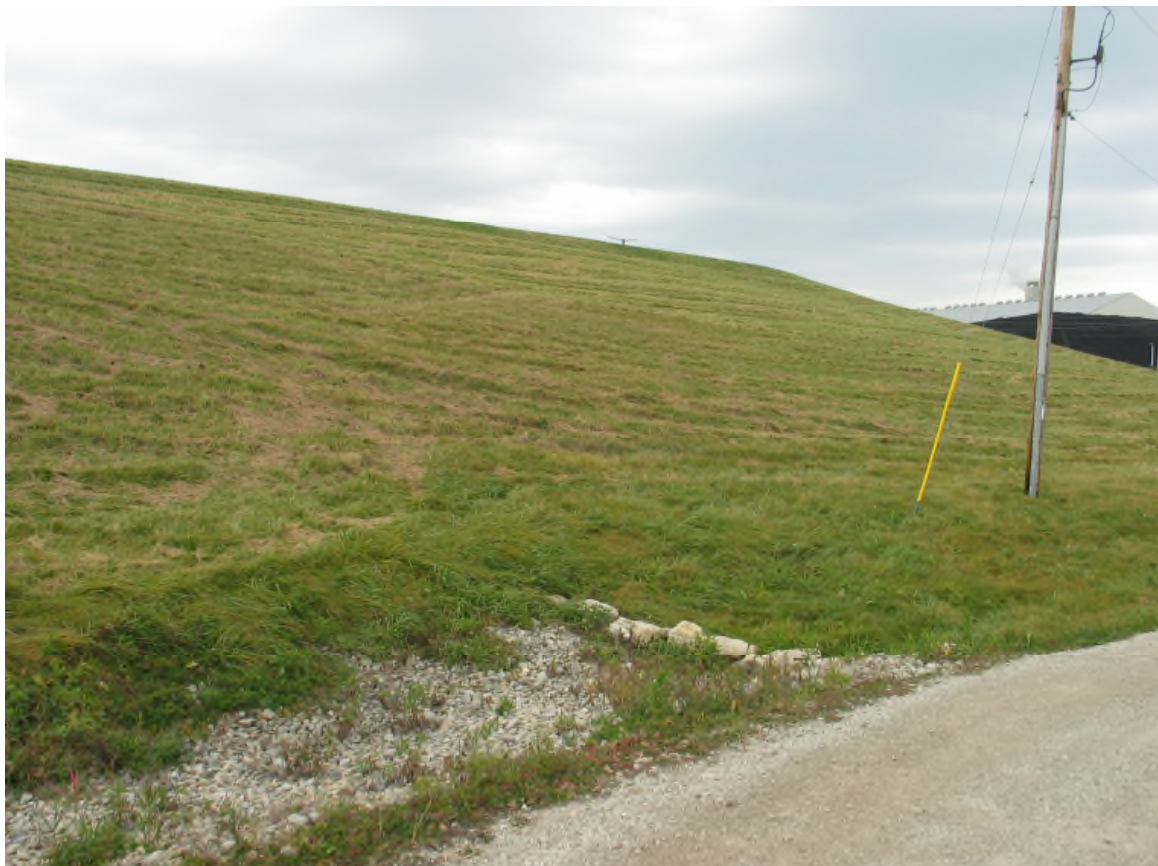
East Side Final Cover (looking north)
